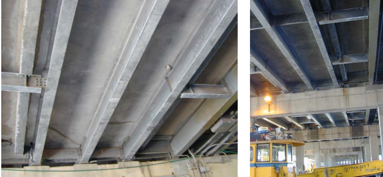
Figure 19. Inverset ™ sections adjacent to existing structure and performing well.
