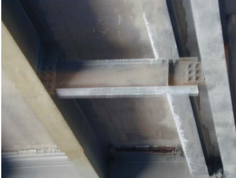
a) Connection with existing and new stringers
