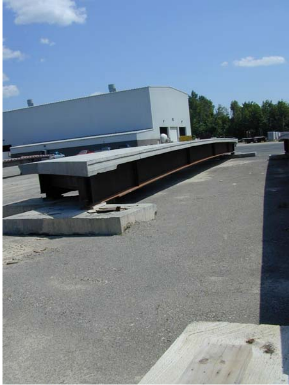
Figure 11. Cambered Inverset TM deck unit.
