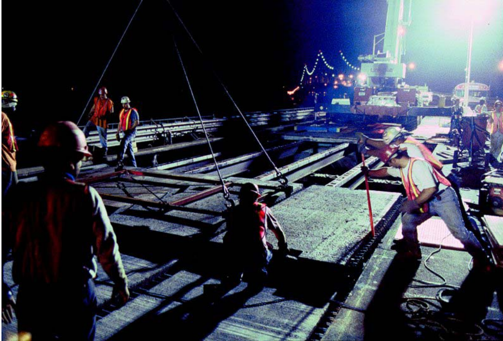
Figure 26. Nighttime construction on the Tappan Zee Bridge.
