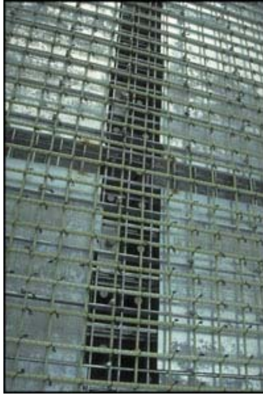
Figure 24. Exodermic TM panel before casting concrete.
