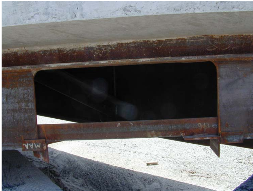
Figure 12. Inverset TM deck unit with provision for utilities.
