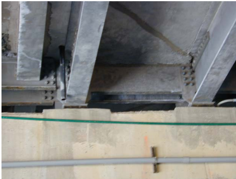
Figure 18. Bearing at a pier.
