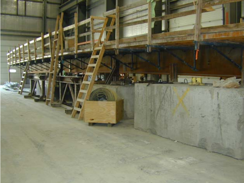
Figure 6. Casting of an Inverset TM deck (at Fort Miller plant).
