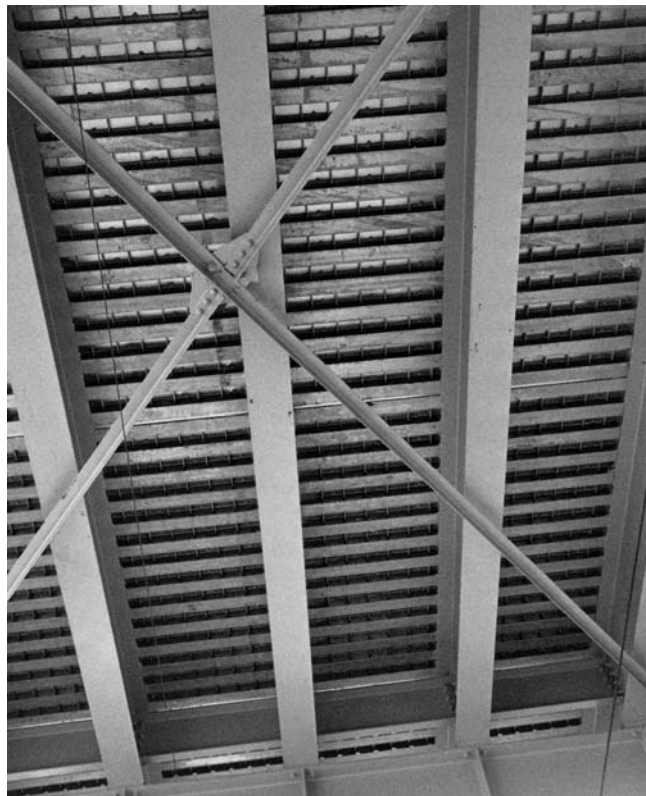
Figure 27. View of an Exodermic TM bridge deck unit (looking from underneath the bridge).
