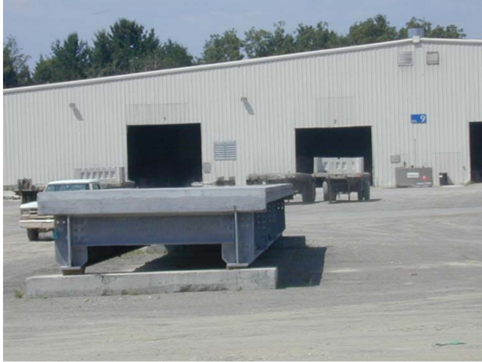
Figure 13. Inverset ™ deck unit with galvanized steel beams.
