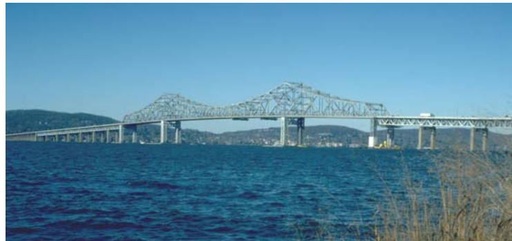
The Tappan Zee Bridge
