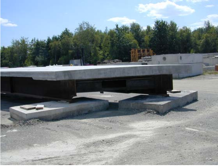
Figure 9. Inverset TM deck unit stored at the precast plant – cross section.
