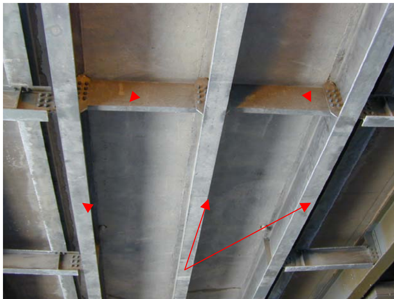
Figure 16. Inverset ™ section installed in the Tappan Zee Bridge.
