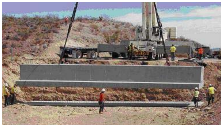
Figure 2.1.3. Photos of Precast Abutment Placement
