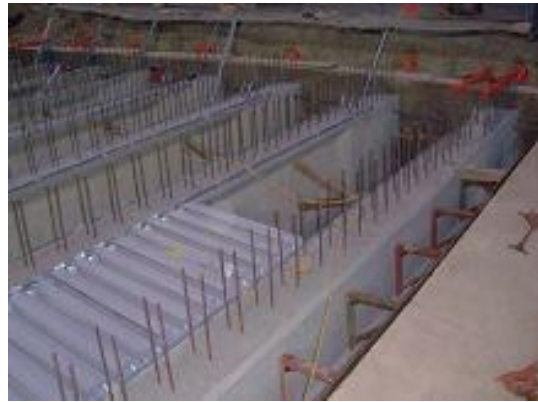
Figure 2.3.3. Photo of Stay-in-Place Metal Deck Form
