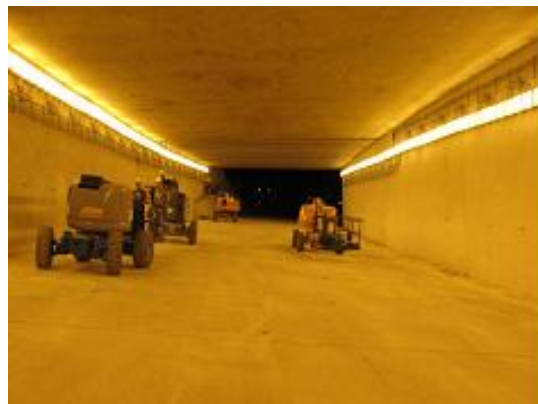
Figure 2.3.4. Photo of Construction Completion
