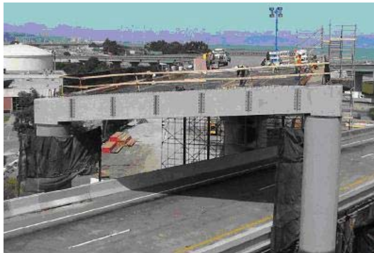
Figure 2.2.8. Completed Concrete Bent Cap
