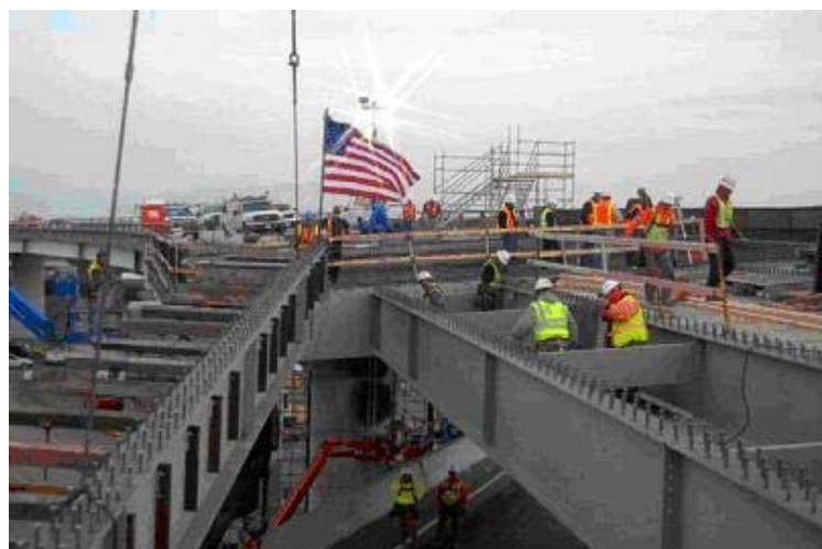
Figure 2.2.9. Last girder installed at the jobsite
