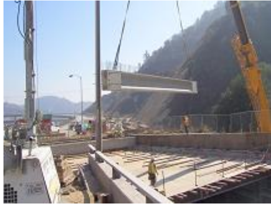
Figure 2.3.2. Photo of Girder Placement
