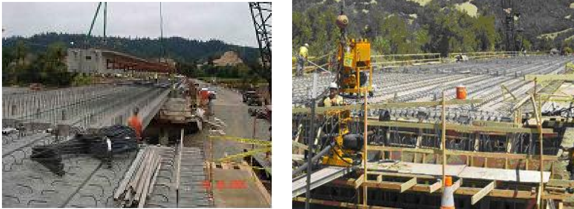
Figure 2.4.5. (b) Construction Photos
