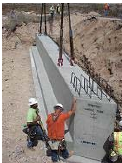
Figure 2.1.2. Photos of Precast Abutment Placement
