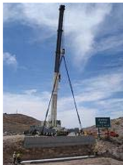
Figure 2.1.2. Photos of Precast Abutment Placement
