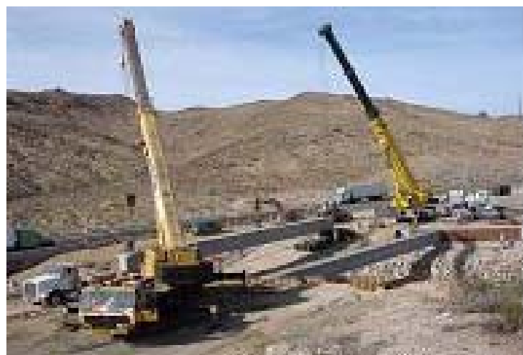
Figure 2.1.4. Photos of Precast Girders Placement
