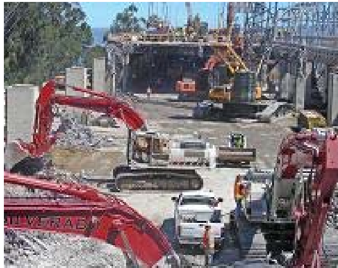
Figure 3.1.1. Photo of Bridge Demolition
