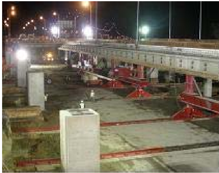
Figure 3.1.2. Photo of New Bridge Roll-in
