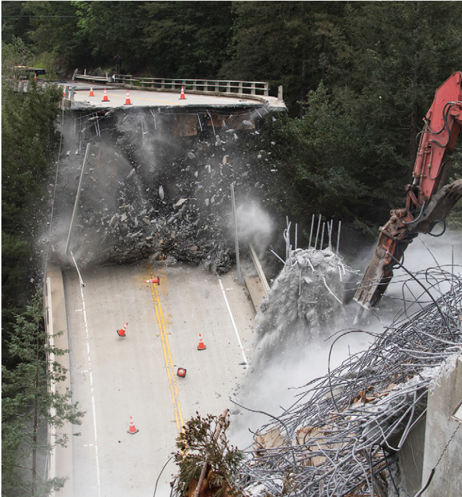
Crews demolished the Pfeiffer Canyon Bridge in March following torrential rains in February that damaged the span. Its replacement is expected to open in mid to late September, using 15 steel girders being constructed in Vallejo, bottom right. Each girder is 63 feet long and weighs 56 tons. They will be connected on site, then rolled into place across the canyon using strategically placed winches and cables.
