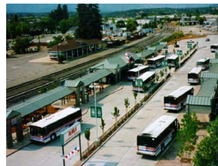
RABA'S Intermodal Facility
