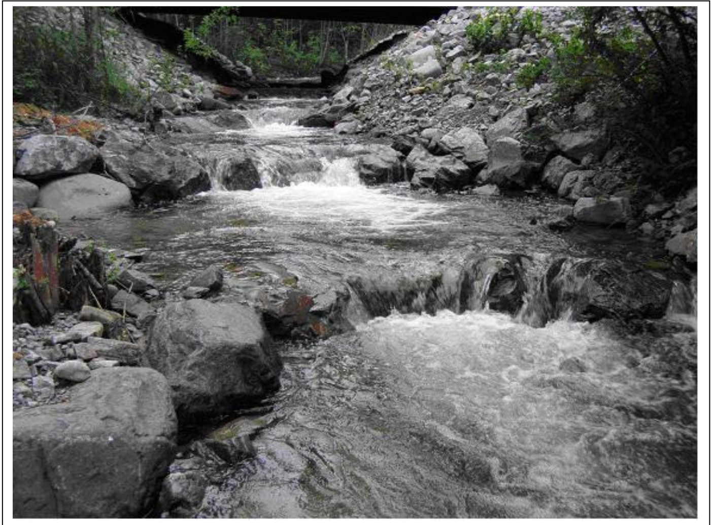
Figure 4. Fish Weir Example
