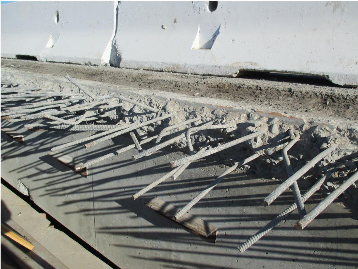
**Figure 6-13. Sawcut Line and Reinforcement Preservation for Widening, Sacramento**
