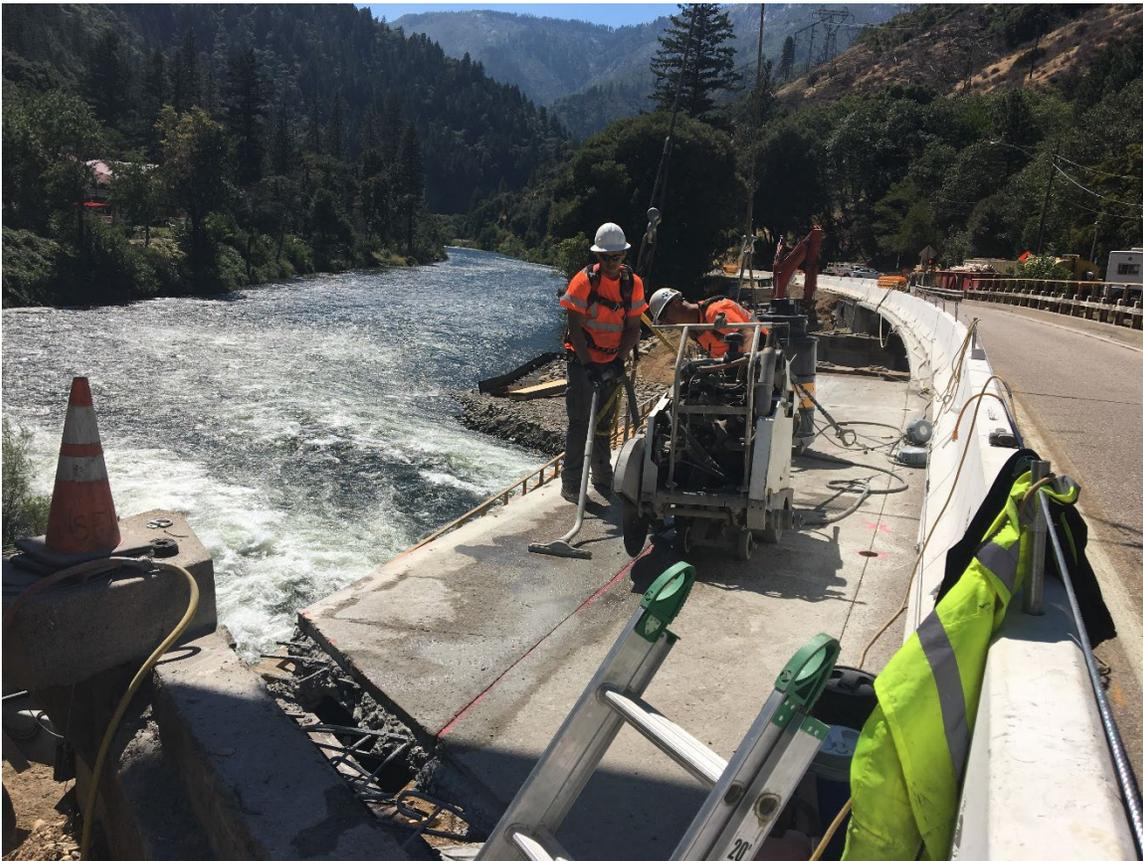
**Figure 6-8. Sawing Deck for Removal, Yellow Creek**
