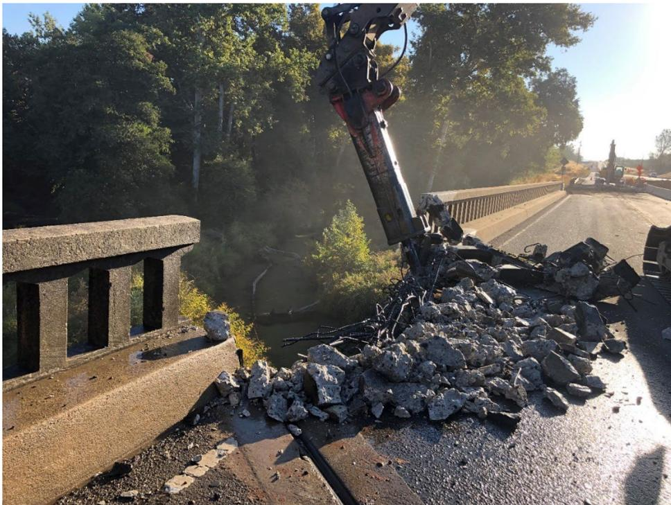
**Figure 6-7. Barrier Rail Removal, Dry Creek**
