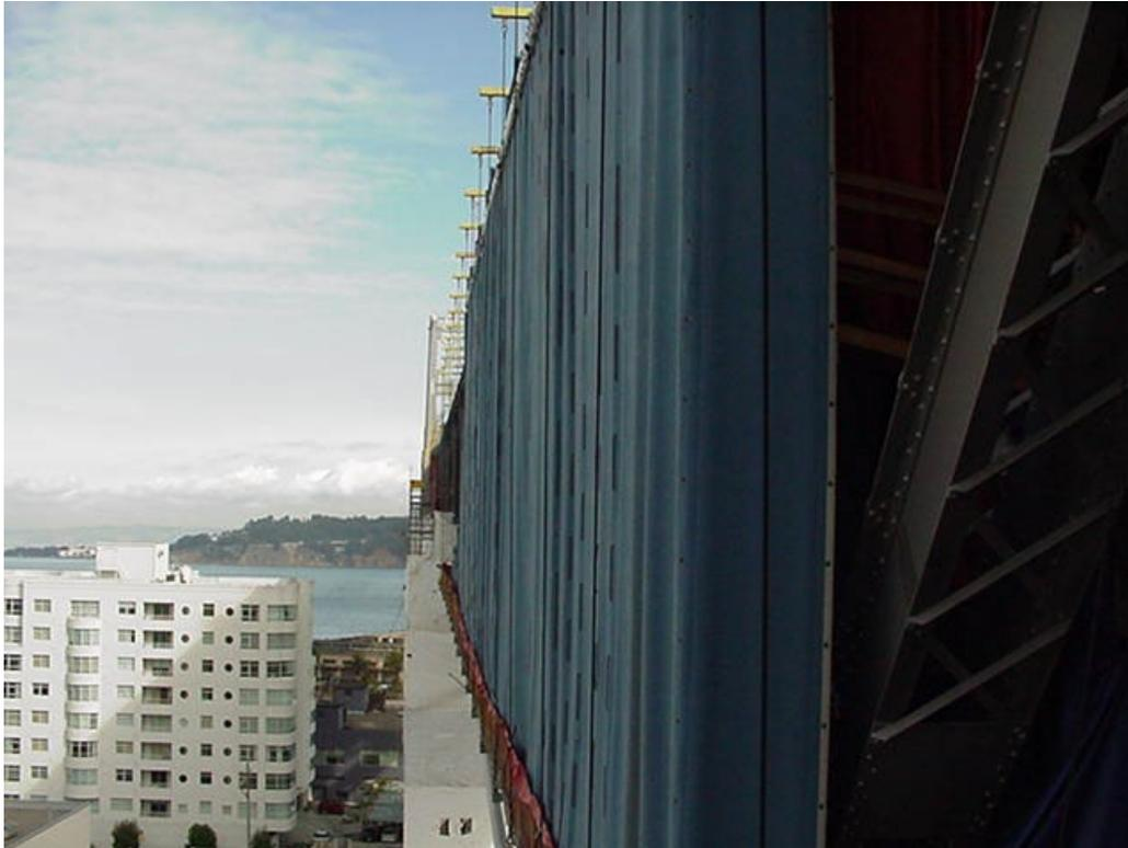
**Figure 7-14. Sound Control Blanket on the Continuous Truss of Bay Bridge**
