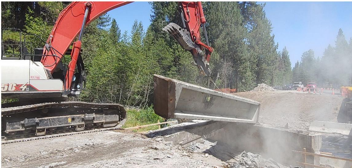
**Figure 4-4. Precast Girder Removal with Excavator, Hat Creek**
