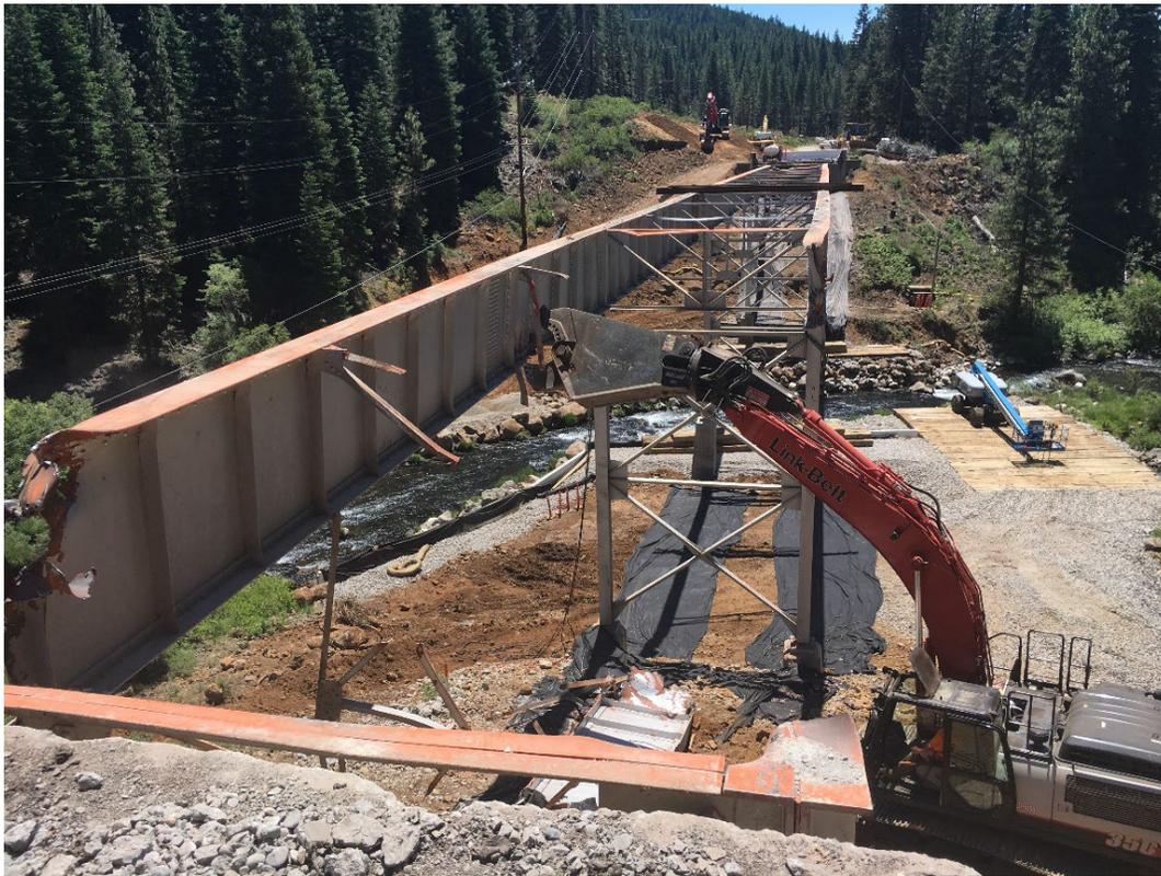
**Figure 6-17. Excavator Mounted Hydraulic Shear Removing Steel Girder, Hamilton Branch**
