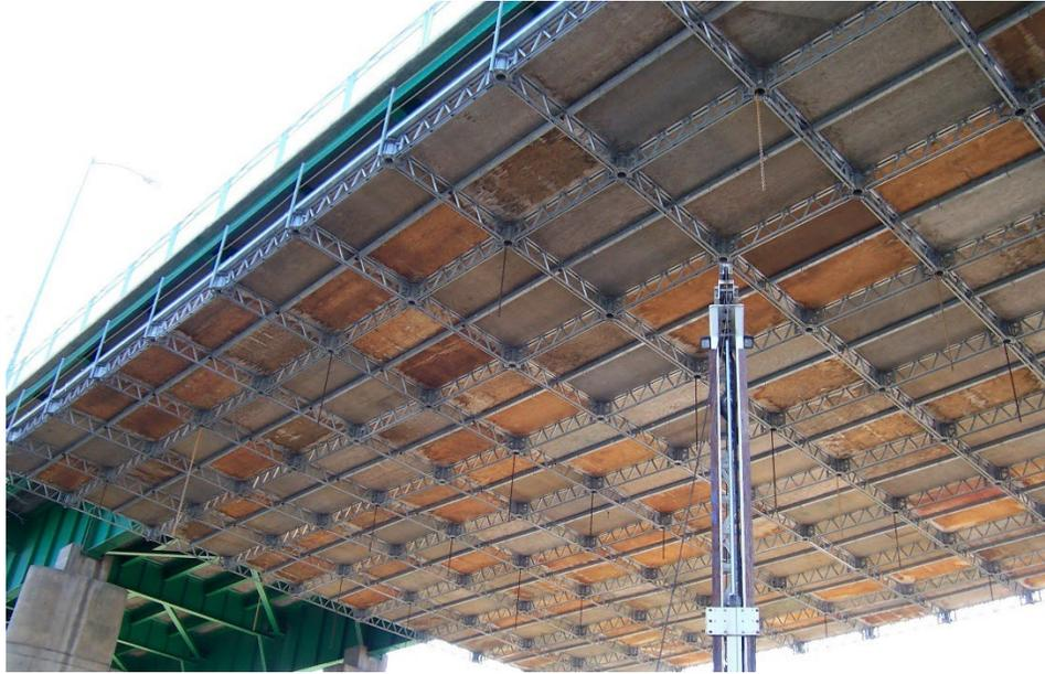
**Figure 5-3. Suspended Scaffolding over River Span, Marysville**
