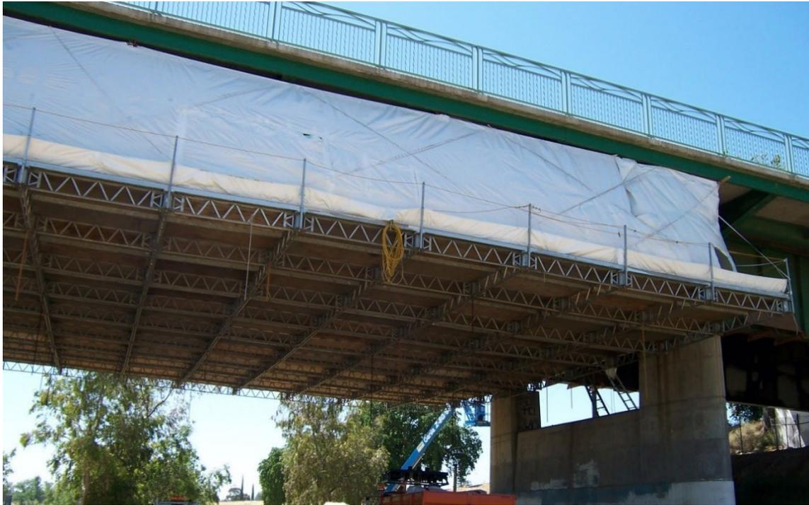
Figure 7-8. Containment System and Work Platform, Feather River
