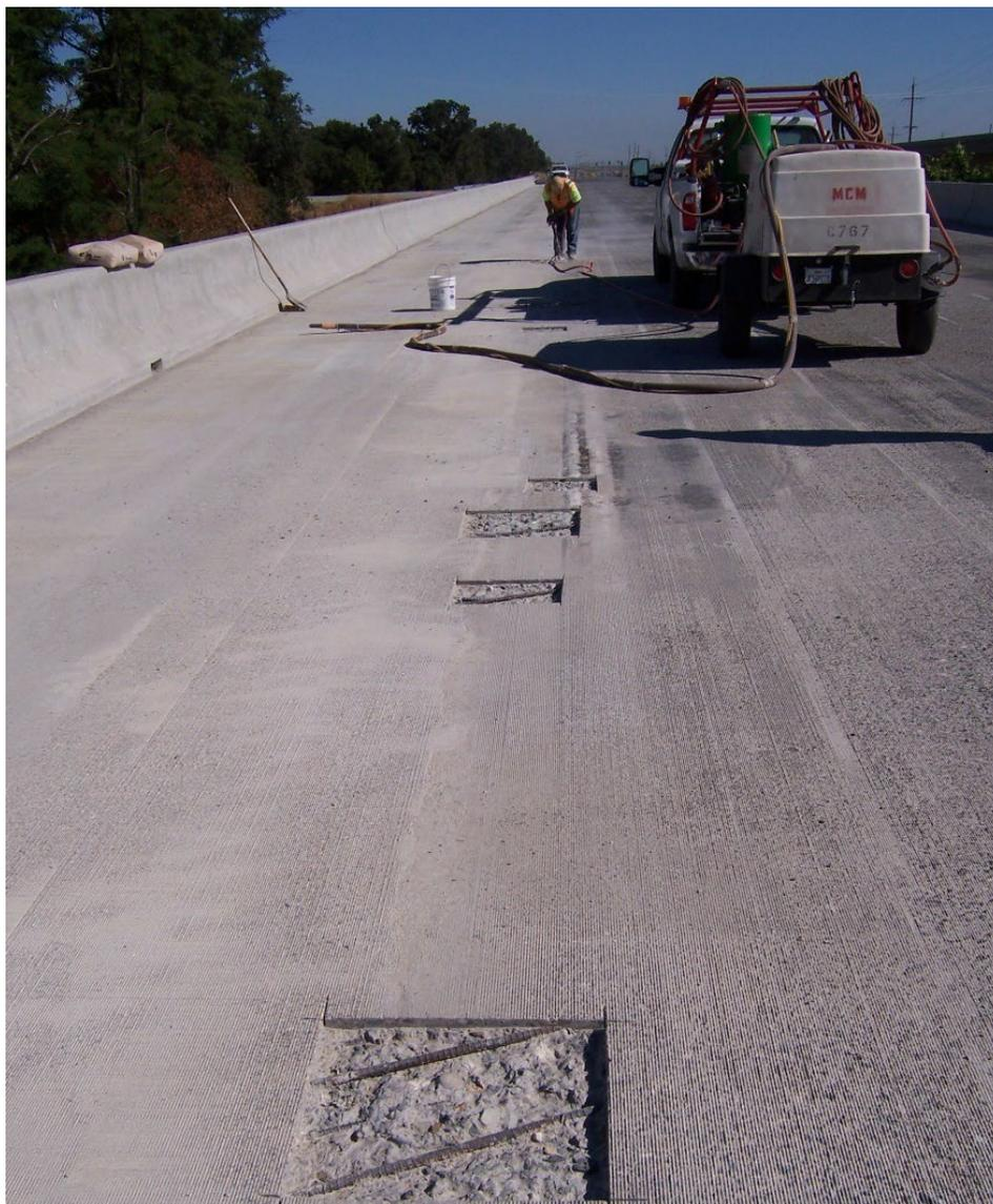
**Figure 6-14. Unsound Concrete Removed for Repair After Asphalt Surfacing Removal**
