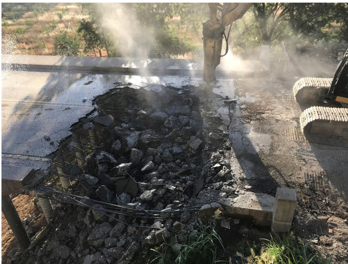
**Figure 6-11. Slab Deck Removal, Simmerly Slough**
