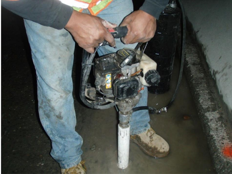
**Figure 6-15. Coring Drainage Hole Through Deck**
