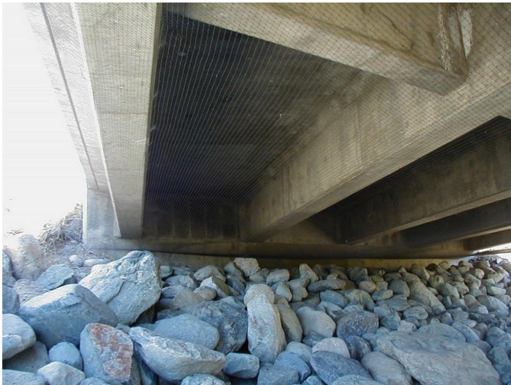
**Figure 7-12. Bird Netting Installed Prior to Demolition**
