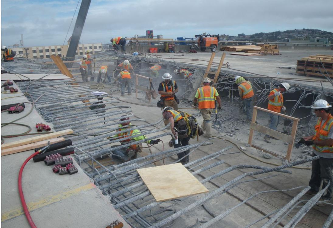
**Figure 8-2. Workers Removing a Portion of a Hinge, San Francisco**
