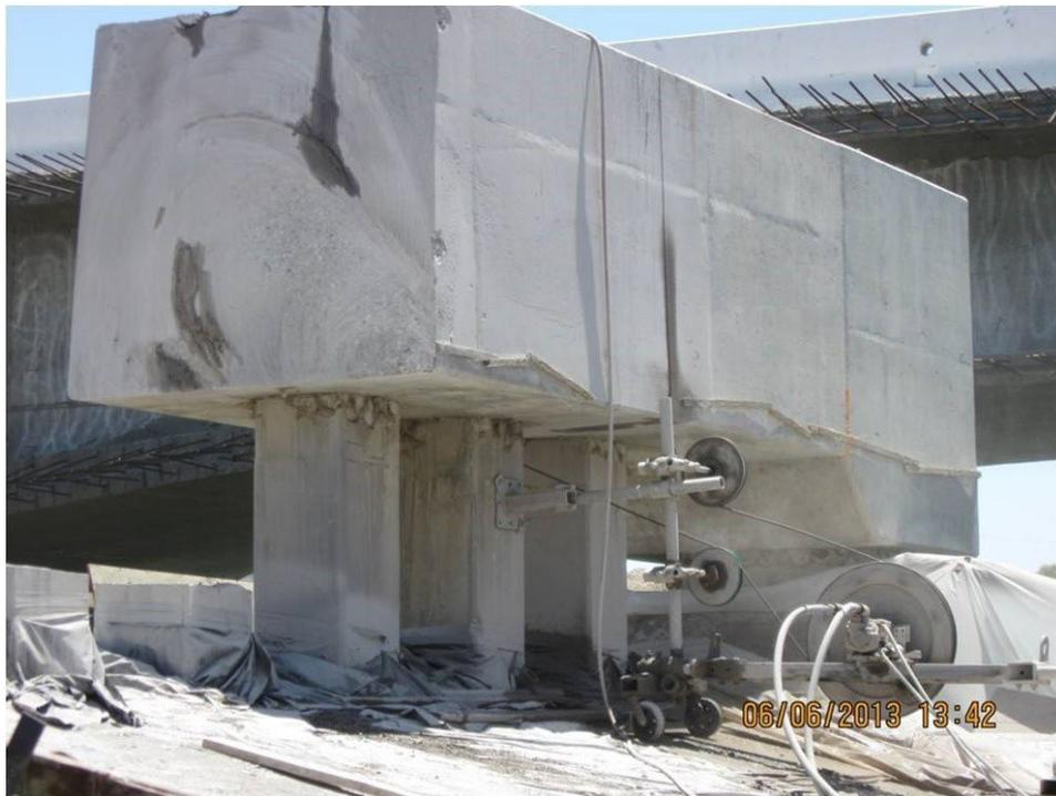
Figure 3-8. Diamond Wire Saw, Colorado River
