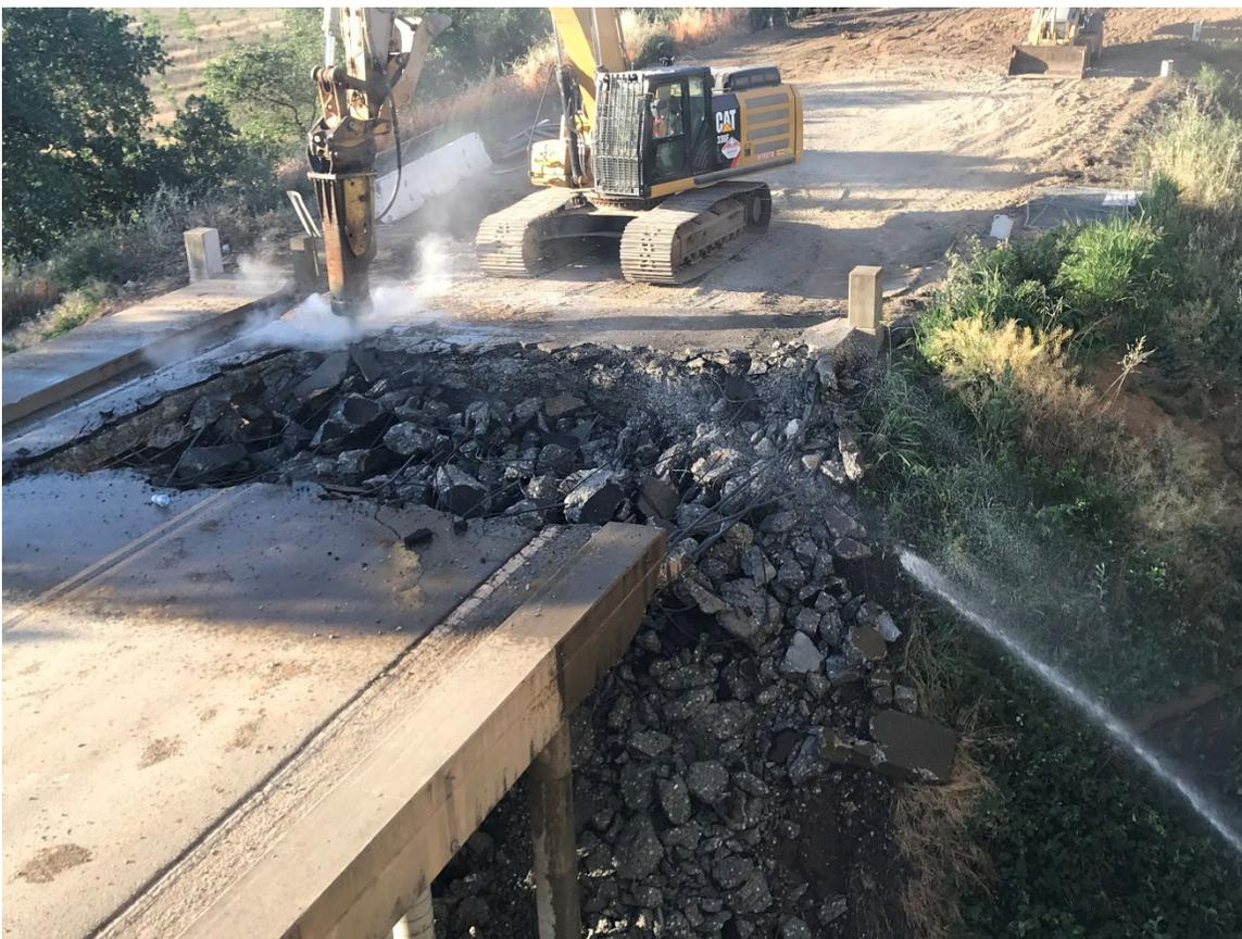
Figure 7-7. Water Applied to Control Dust, Simmerly Slough
