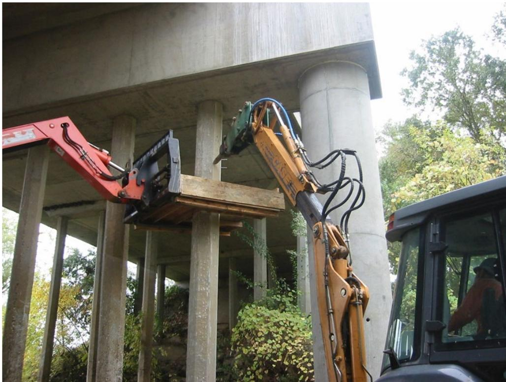
**Figure 7-2. Debris Containment Platform, Honcut Creek**
