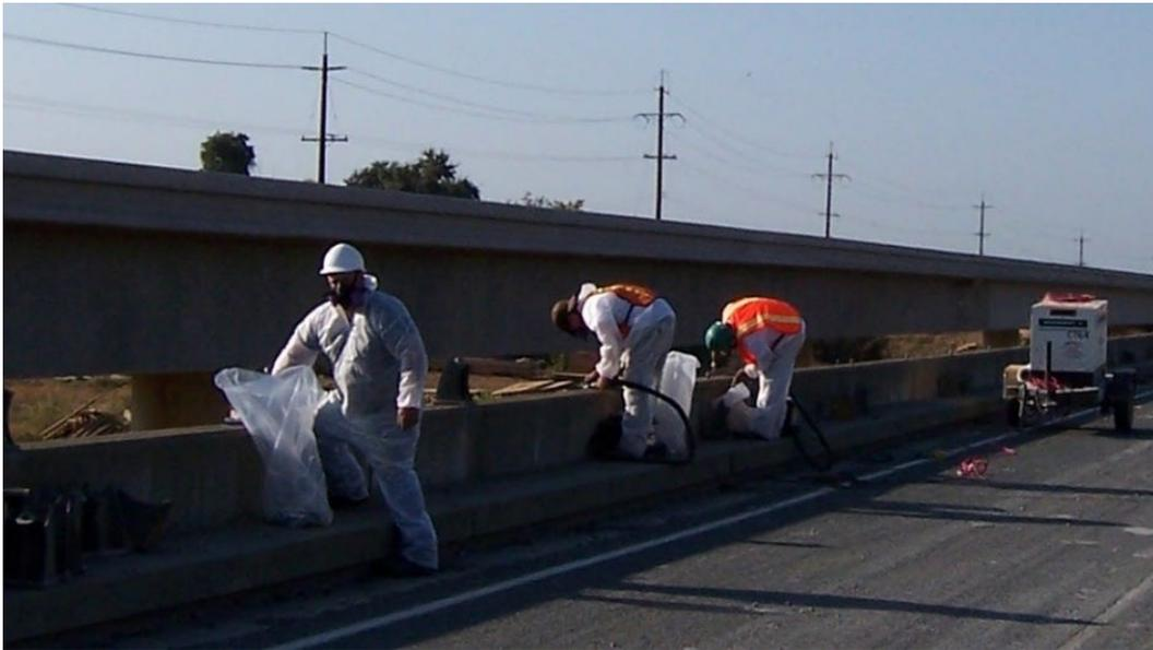
**Figure 6-4. Asbestos Shim Removal**
