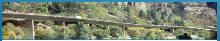
Viaduct example on I-70 in Colorado. Colored concrete matches local rock. Vegetation around viaduct columns visually integrates structure.
