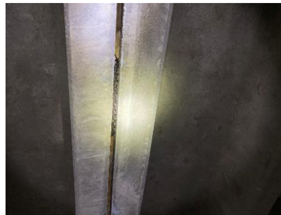
Photo 16. Habitat surrounding concrete girder bridge, and the gaps between girders (potentially suitable bat roost habitat), consists of annual grass, agricultural fields (rice) and potential tree roost habitat with dense clusters of leaves and crevices within Yolo Bypass (Location #29). One thousand five hundred Mexican free-tailed bats were counted in one section of the bridge. Taken facing up towards gaps in girders.
