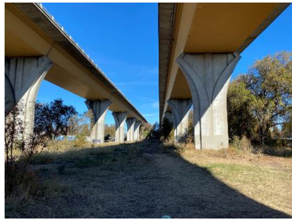
Photo 26. Habitat along steel box bridge with multiple expansion joints and crevices observed along the bridge abutment consists of landscaped lawns, mowed areas below the bridge, residential and industrial buildings, homeless encampments, and potential tree roost habitat along the Sacramento River and urban street trees with dense clusters of leaves and crevice (Location #46). Taken facing northeast.
