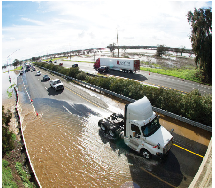
Highway 99, in southern Sacramento County, was inundated earlier this year. Caltrans District 3, which takes in Sacramento and a swath of the Sierra, absorbed $129.6 million in weather-related damage.
