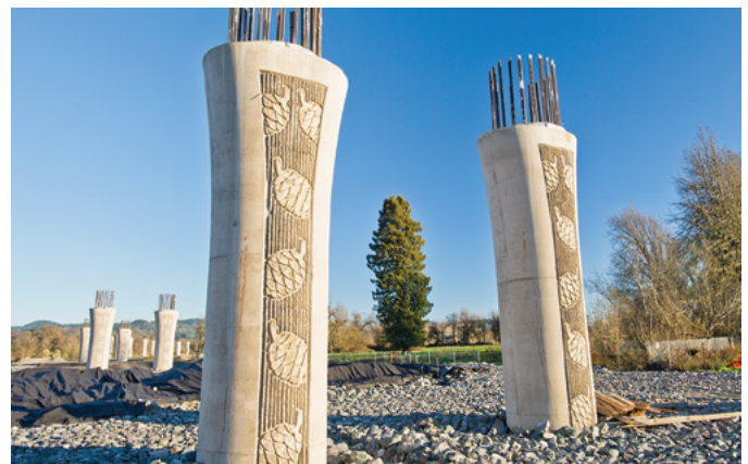
These columns, or bents, rise over 20 feet to support the 1.1 mile viaduct. In all, 64 of these columns support the viaduct's roadway.
