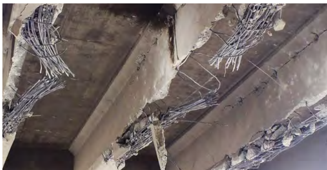
The Walters Road overpass on Interstate 5 south of Yreka sustained massive damage in 2012 after being struck by a high load. At right, the overpass is being removed prior to replacement.
