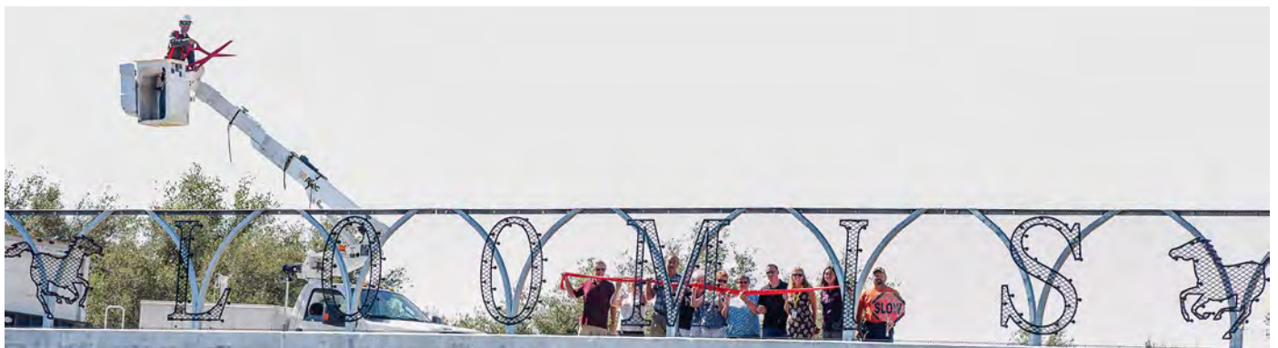
In the town of Loomis, along I-80, Loomis Chamber of Commerce members, town officials, Caltrans staff and neighbors held a ribbon cutting for the town’s new Western-themed artwork on the Horseshoe Bar Road crossing.
