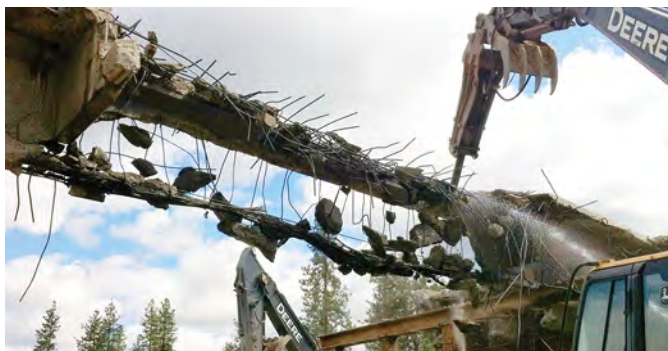
The Walters Road overpass on Interstate 5 south of Yreka sustained massive damage in 2012 after being struck by a high load. At right, the overpass is being removed prior to replacement.
