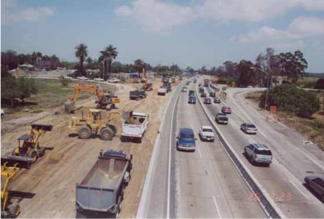
Figure 2. Around-the-clock construction operations with counter-flow traffic divided by MCB
