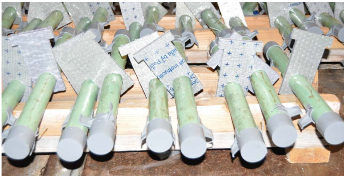
Figure 330-2: Dowels with end caps, support chairs, and foam inserts
