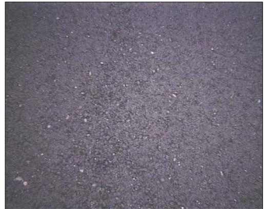
New tight DGAC surface. Application rates of more than 0.06 gal/sq yd could result in slick surface. Not suitable for fog or rejuvenator seal on high speed facilities.
