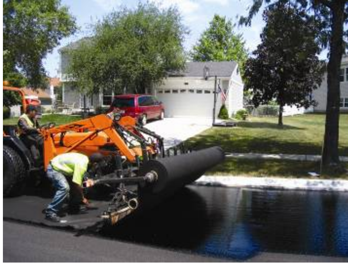
Figure 12-10 Tractor Mount Application of Fabric
