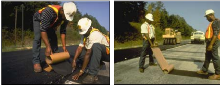
Figure 12-5 Application of Composite Membranes
