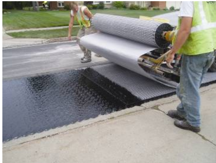
Figure 12-13 Composite Paving Grid Installation
