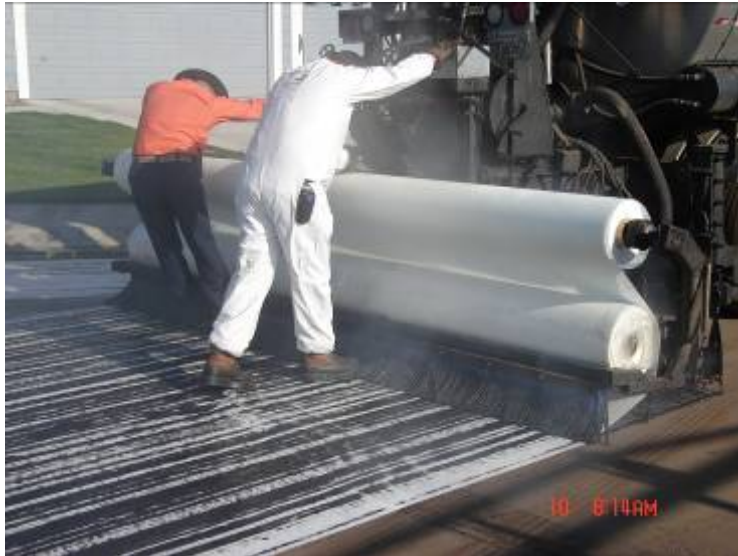
Figure 12-11 Truck Mount Application of Paving Mat
