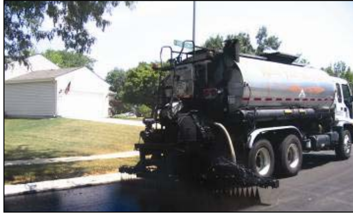
Figure 12-9 Interlayer Binder Application
