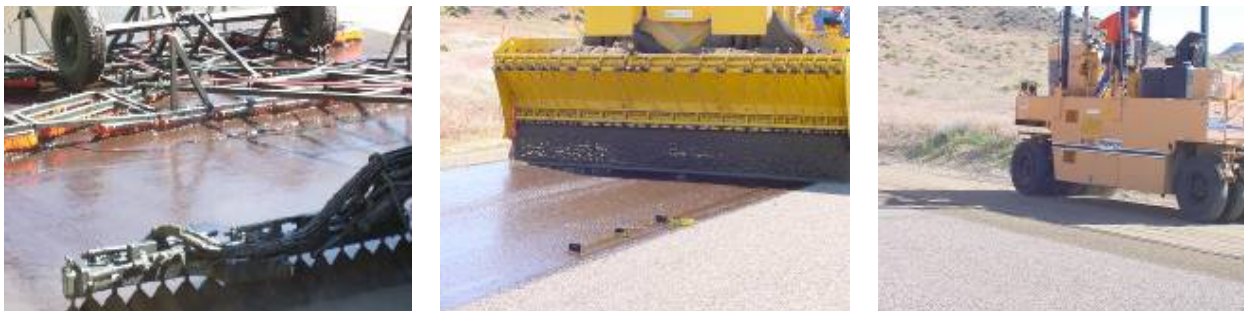
Figure 12-17, 18, 19 Scrub Seal Construction
