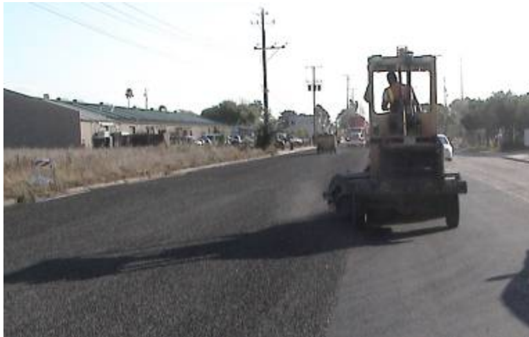
Figure 12-16 Chips Applied and Sweeping Edge for 2 nd Pass
