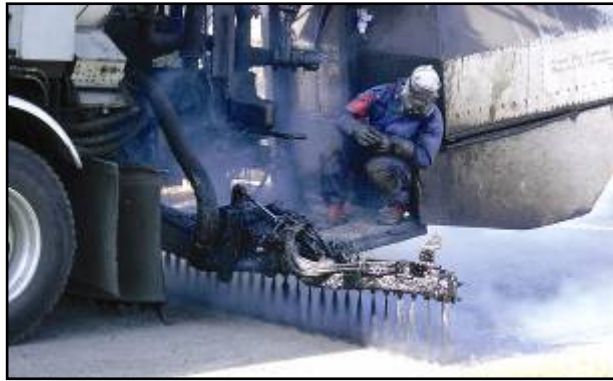
Figure 12-14 Asphalt Rubber Binder Being Applied
