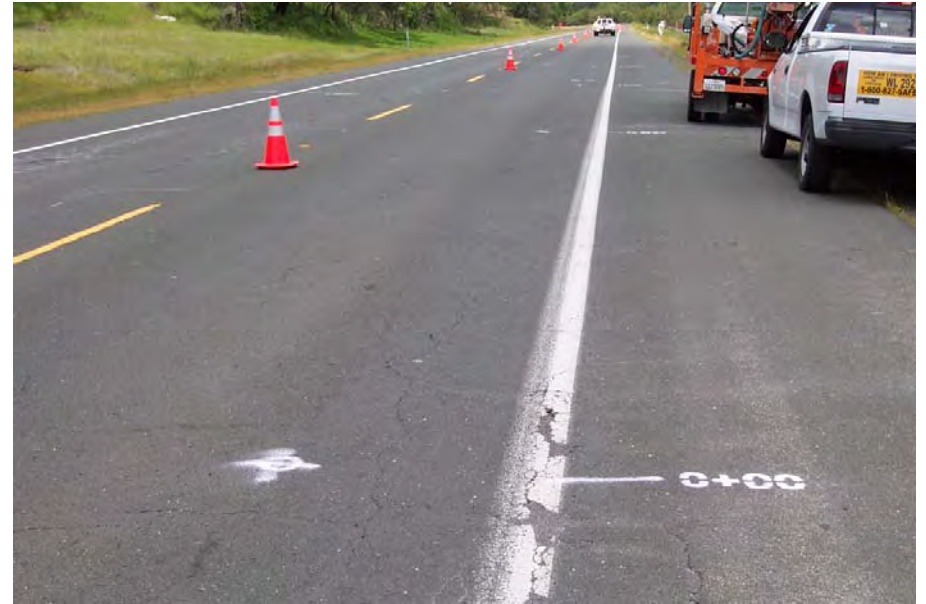
Pavement Condition within PES 4
