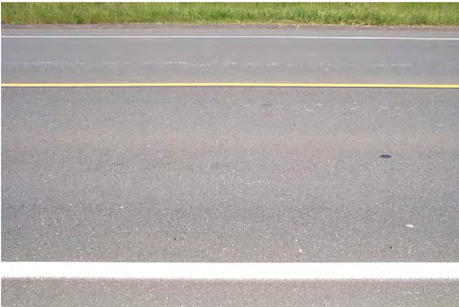
Pavement Condition within PES 1
