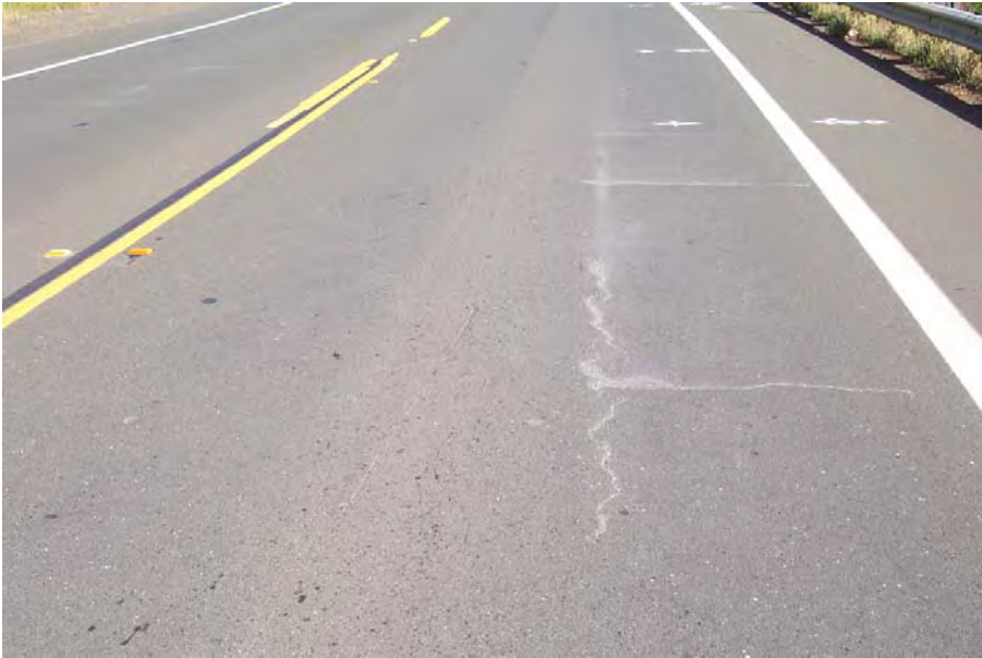
Pavement Condition within PES 2
