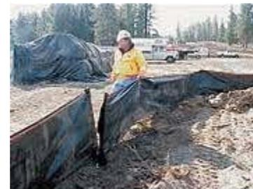
Upon inspection, it was determined that this silt fence was installed incorrectly.
