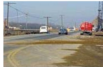
Visibly tracked sediment must be removed from roadways.
