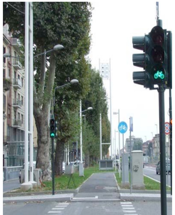
Figure 9 Bicycle signal head assigns ROW to through bicycles while left turning drivers face a red arrow.
