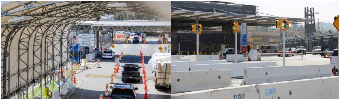
Private vehicle border crossing at Otay Mesa. Left: cones divide vehicle queues. Right: cement blockades divide vehicle queues. The focus is on security, not mobility or economic development.
