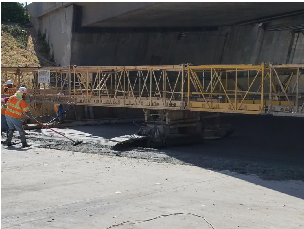
Photo of Castillo Street concrete pour nearing completion this morning.
