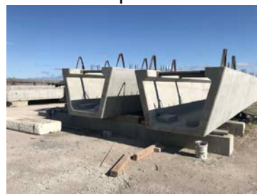
Photos of pre-cast girders, also called “California Bath Tub Girders”—each 125ft long and weighing 200k lbs.
