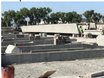
Photos of pre-cast girders, also called “California Bath Tub Girders”—each 125ft long and weighing 200k lbs.
