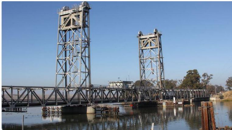
Caption: SR-160 Three Mile Slough Bridge (December 2018)
