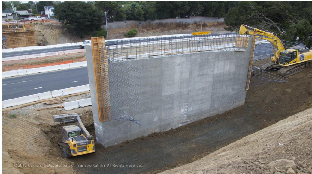
Large equipment work on early bridge infrastructure. (Caltrans Photography, August 8, 2017)
