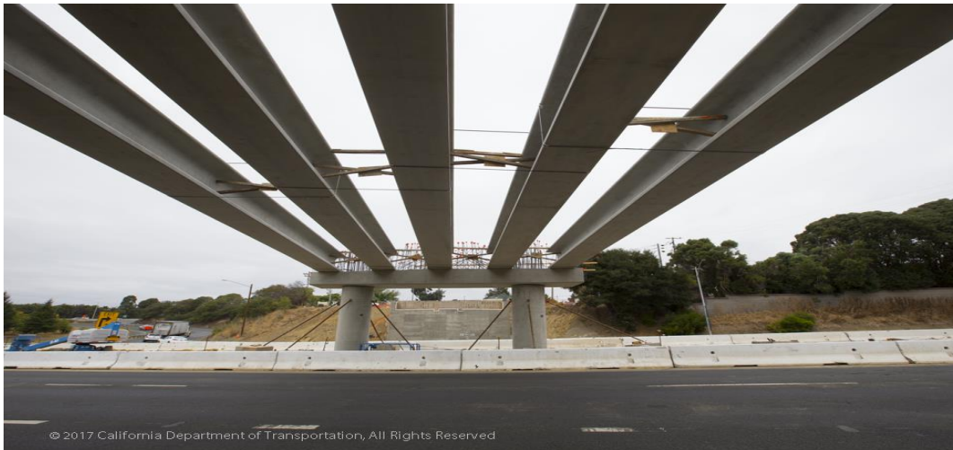
Early installation of girders across I-780 (Caltrans, Photography, September 13, 2017)
