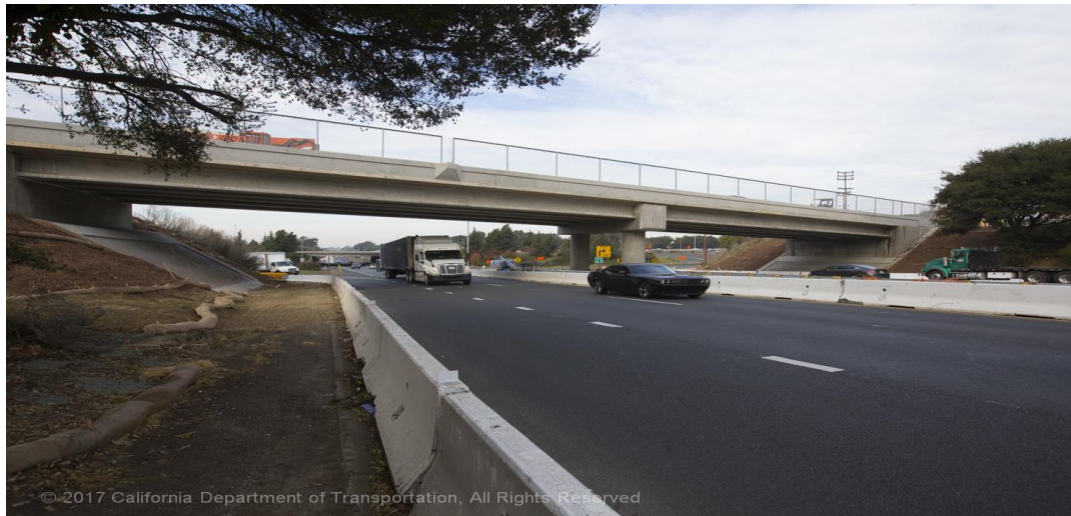
New I-780 Laurel Street Bridge in Vallejo, CA (Photos by Caltrans Photographer John Huseby)
