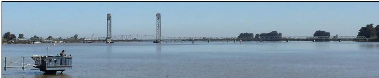
The first project will maintain and preserve the steel structural members of the Rio Vista Bridge (No. 23-0024) on State Highway 12 over the Sacramento River by cleaning and painting all steel surfaces.
