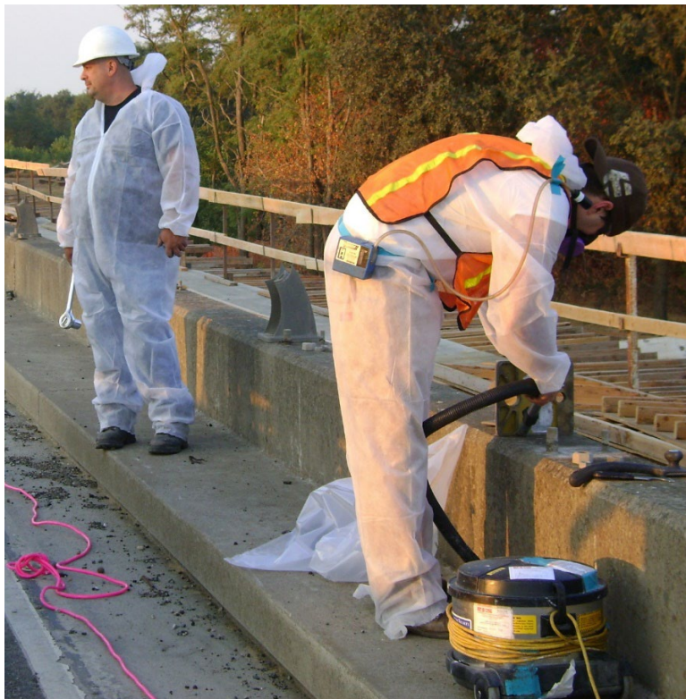
Figure 7-6. Asbestos Shim Removal from a Bridge Rail
