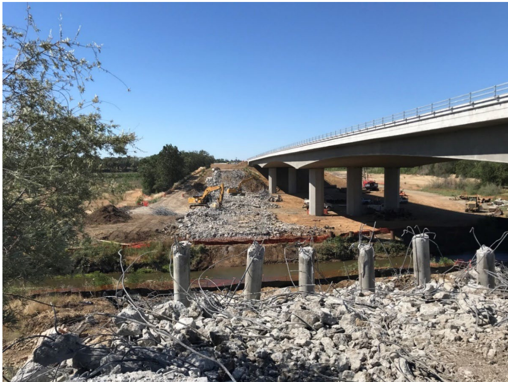
Figure 7-4. Debris Processing with Water Pollution BMPs in Place, Simmerly Slough
