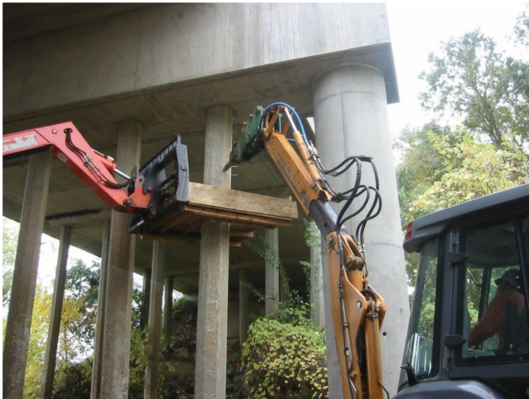
Figure 7-2. Debris Containment Platform, Honcut Creek
