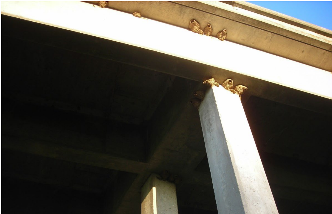
Figure 7-10. Common Location for Swallows' Nests on Bridges
