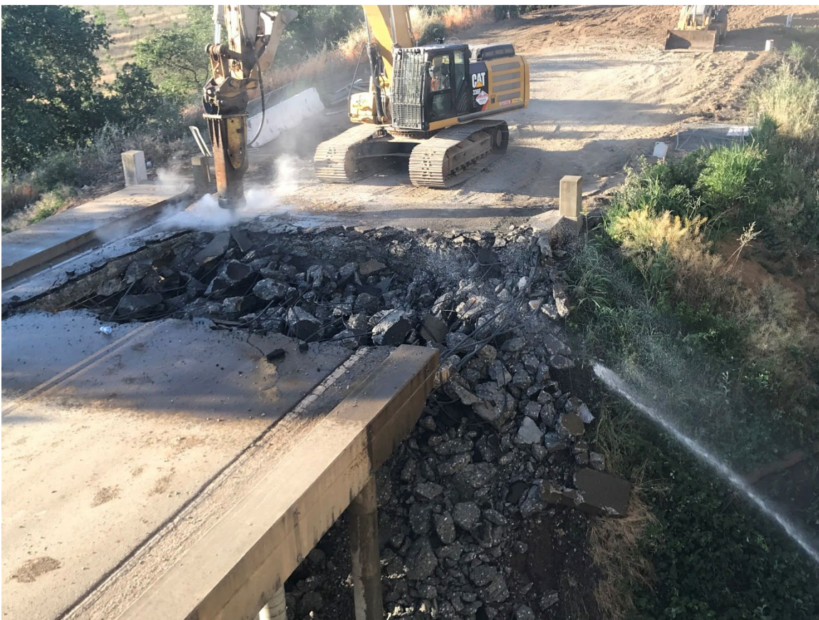
Figure 7-7. Water Applied to Control Dust, Simmerly Slough
