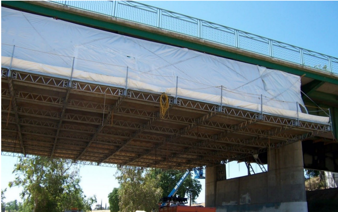
Figure 7-8. Containment System and Work Platform, Feather River
