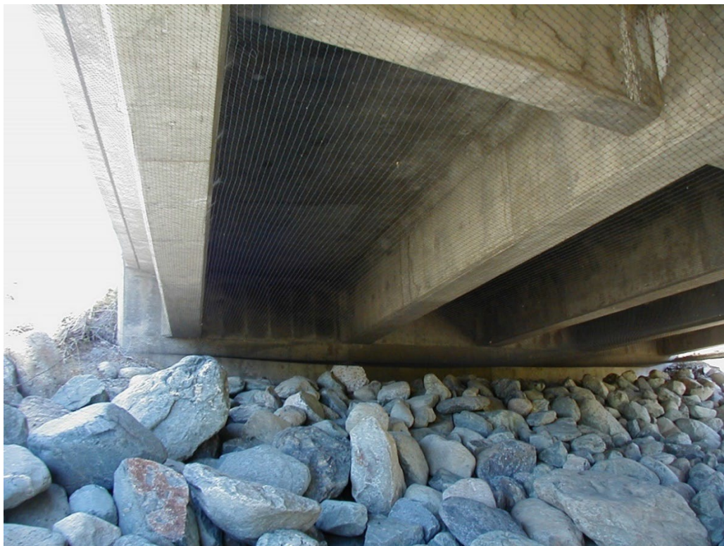
Figure 7-12. Bird Netting Installed Prior to Demolition
