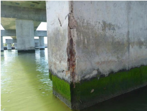
Photos from Bridge Inspection Report: Existing Column Conditions
