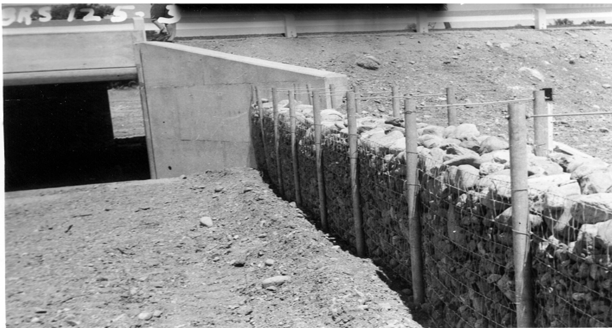
Figure C5-8: Rock filled double pipe and wire fence, Dry Creek, Lake County. Courtesy, Steve Hg, Maintenance and Investigation Office, 4-98.
