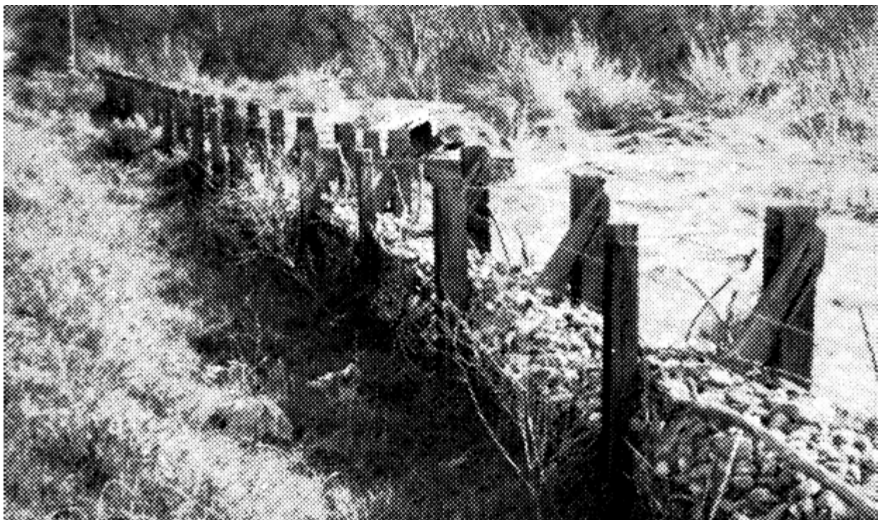
Figure C5-15: Double Row of Fence, rock Filled, District 5, San Benito River Courtesy, Steve Ng, Maintenance and Investigations Office, 4-98.
