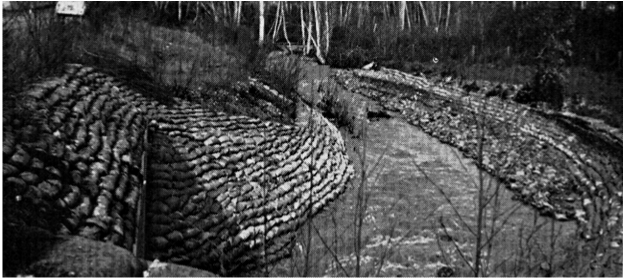
Figure C5-7: Sacked Concrete Slope Protection, District 2, Trinity County,. Courtesy, Steve Ng, Maintenance and Investigation Office, 4-98.
