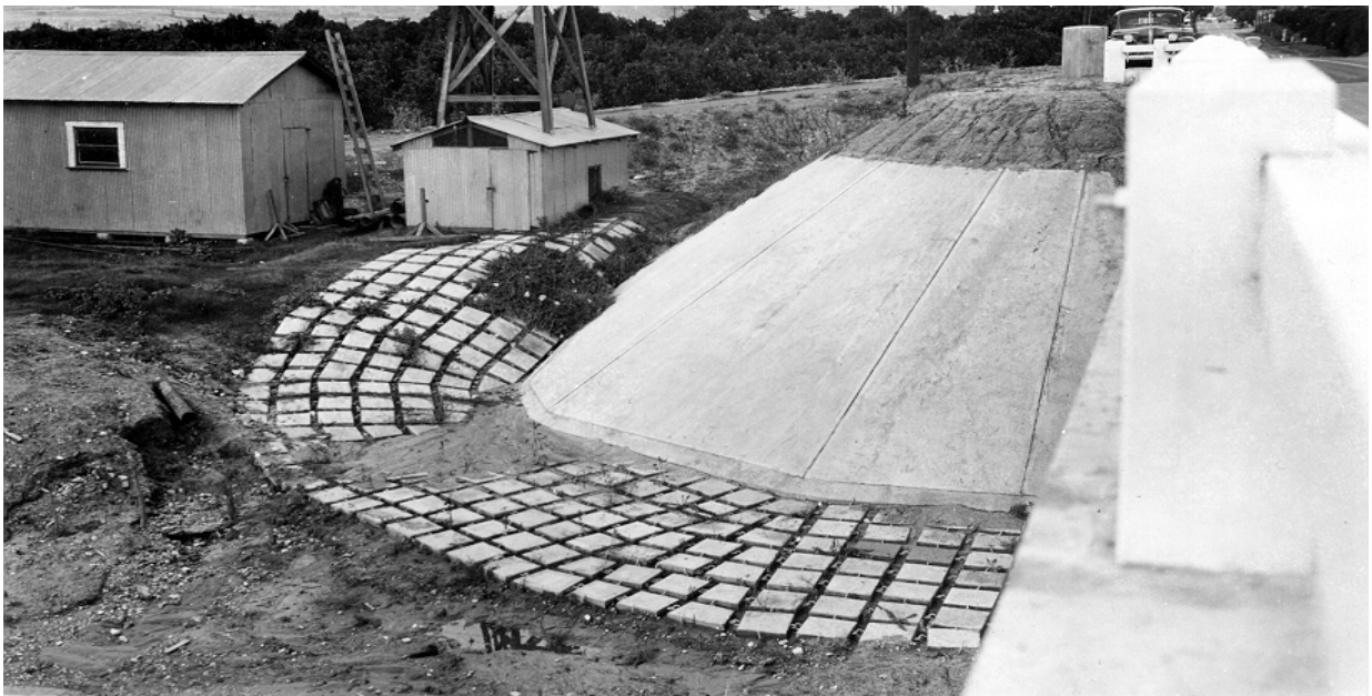
Figure C5-10: PCC Mattress and Concrete Paved Slope Protection Courtesy Steve Ng, Maintenance and Investigations Office, 4-98.
