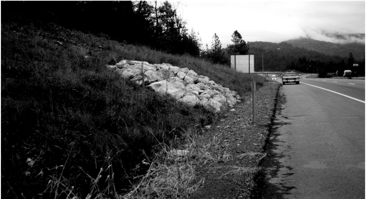
Figure C5.-3: Half-ton RSP, 2-Sha-5, Postmile 50.1. Courtesy, Kathy Coots, Maintenance Supervisor, 2-98.
