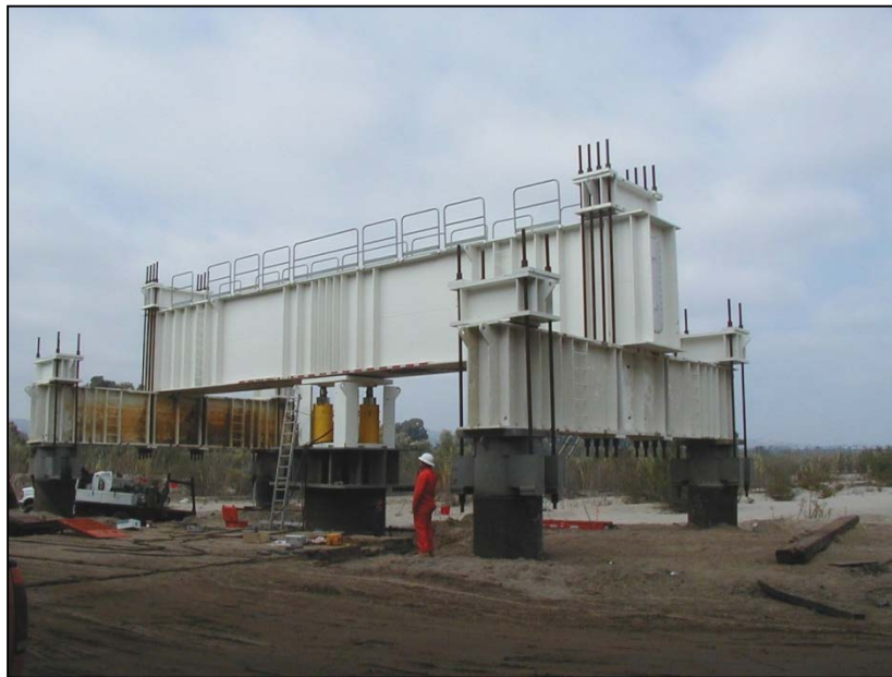
Figure 8-1. Static Pile Load Test (Five-Pile Array).
