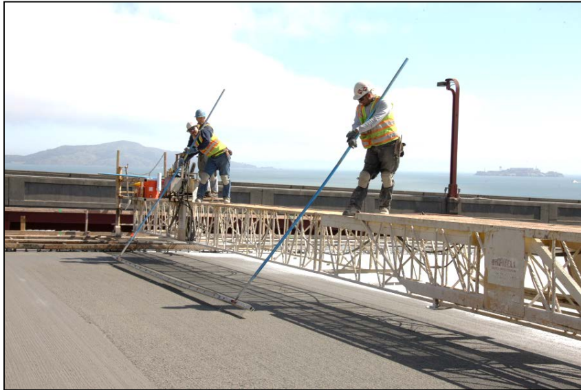
Figure 6.1-6. Longitudinal Tining Typical Process.
