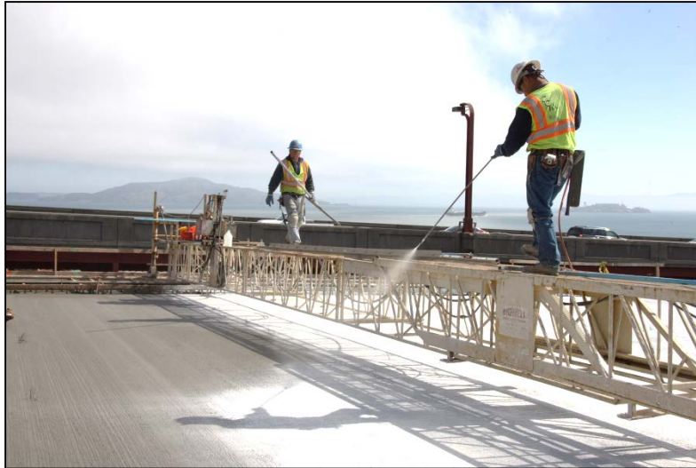
Figure 6.2-1. Applying Spray Cure from a Moveable Bridge Following the Finishing Machine.
