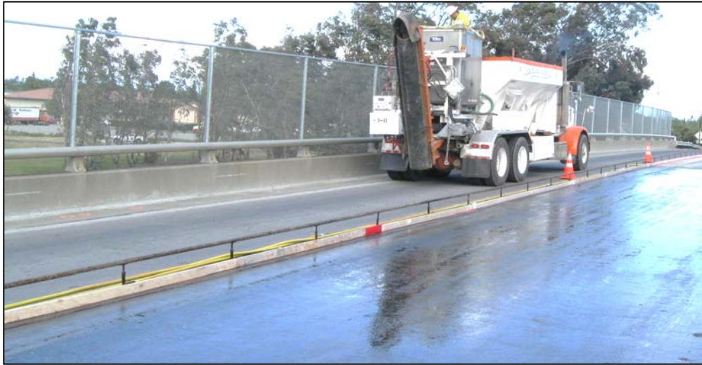
Figure 6.1-4. Typical Grade Rail Setup.
