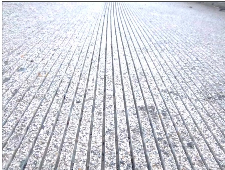
Figure 6.1-7. Close-up of Grooving.
