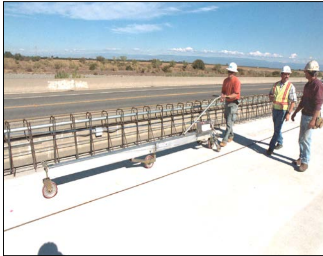
Figure 6.1-1. Smoothness Testing, per California Test 547.
