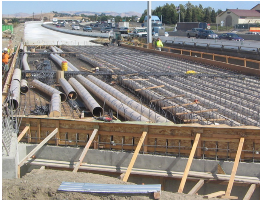
Figure 5-6. Fiber Forms Used for Forming Voided Slab Structure.
