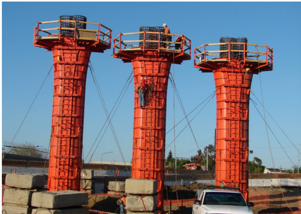
Figure 5-5. Steel Column Forms.
