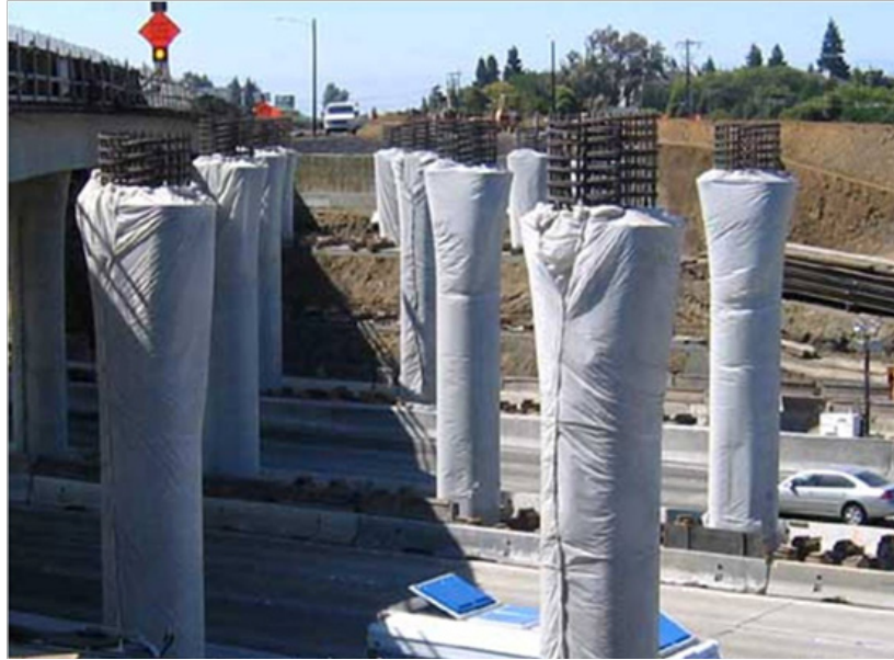
Figure 5-23. Curing Concrete Columns Using Polyethylene Plastic Sheets.
