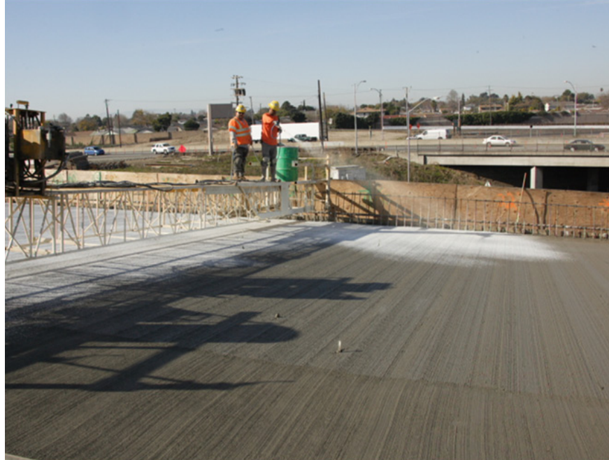
Figure 5-27. Applying Curing Compound Using Power-Operated Spray Equipment.
