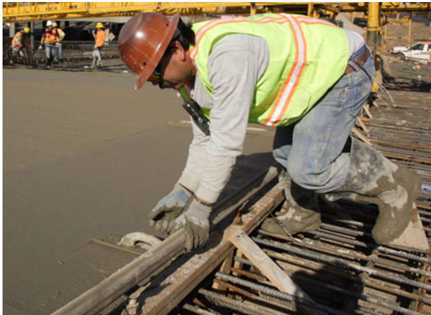
Figure 5-16. Hand Floating a Bridge Deck.
