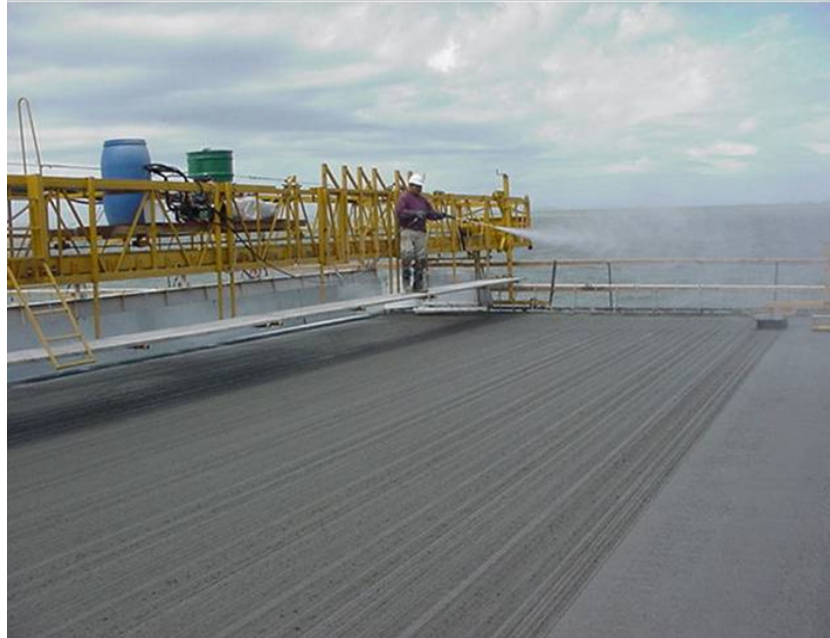
Figure 5-26. Fogging Bridge Deck to Minimize Plastic Cracking.
