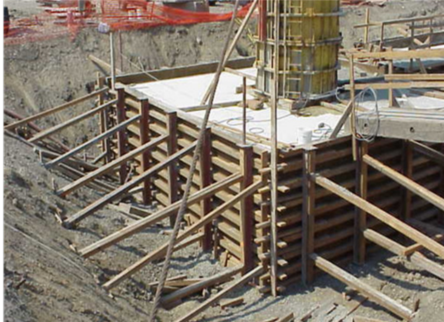
Figure 5-25. Forms-In-Place Curing Method.
