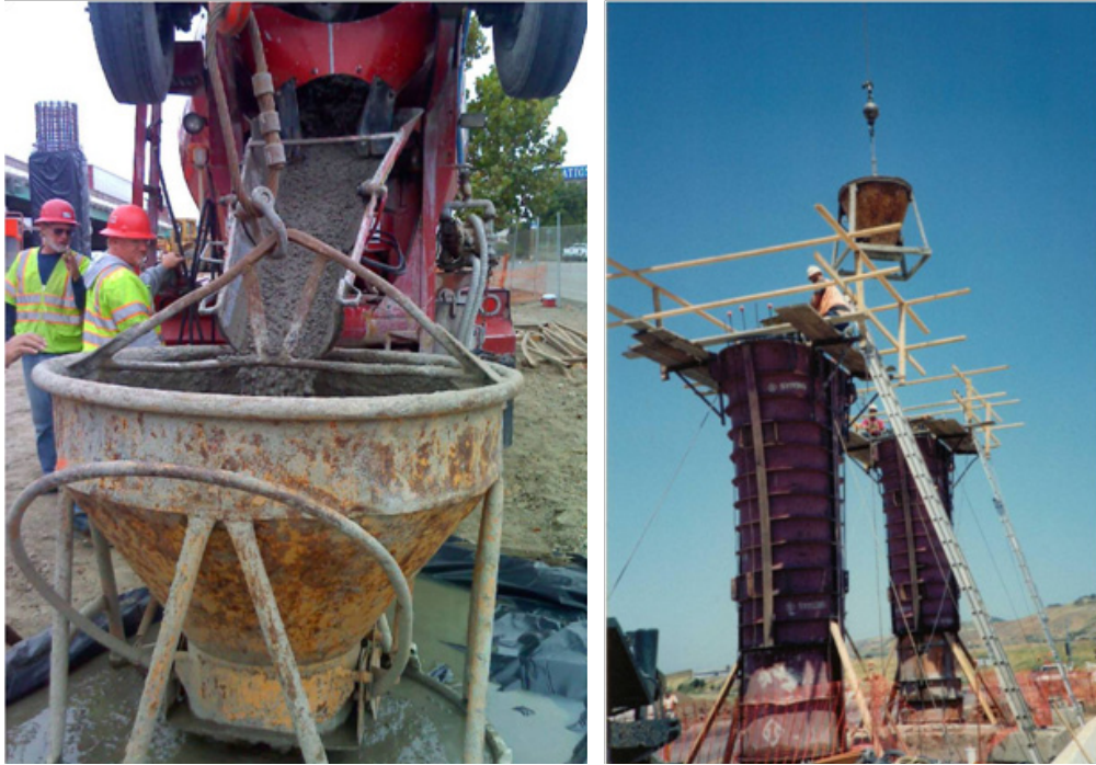
Figure 5-10. Crane and Bucket Method.
