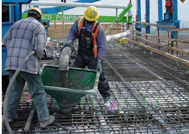
Figure 5-12. Depositing Concrete Using a Drop Chute.
