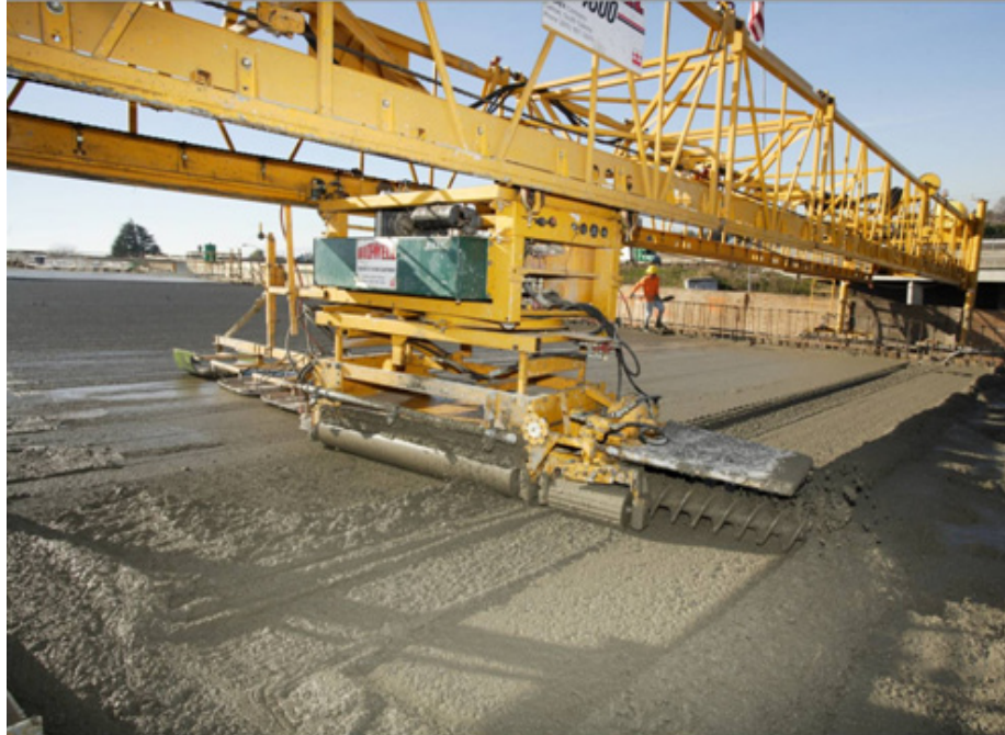
Figure 5-19. Bidwell Concrete Finisher.
