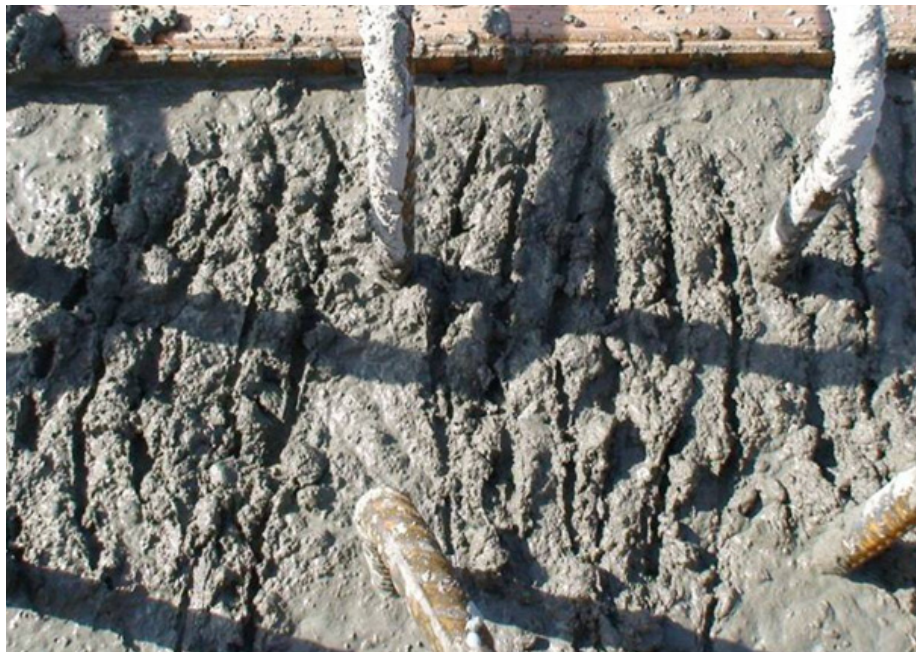
Figure 5-29. Stem Concrete with 1/4 Inch Roughening.
