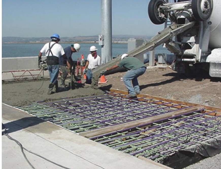
Figure 5-9. Concrete Transit Mixer Truck with Built-In Delivery Chute.
