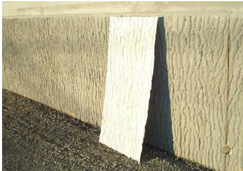
Figure 5-4. ABS Panel Liner and Resulting Wall.
