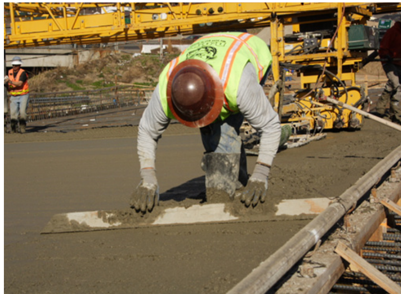
Figure 5-15. Striking Off Bridge Deck Concrete.
