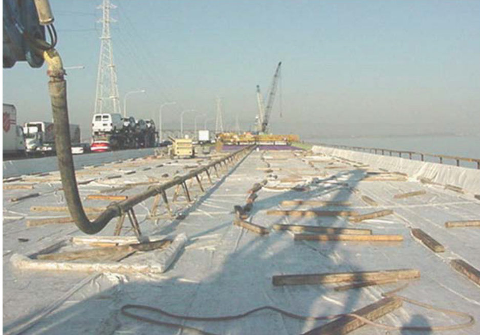
Figure 5-13. Slick Line Used to Deliver Concrete.
