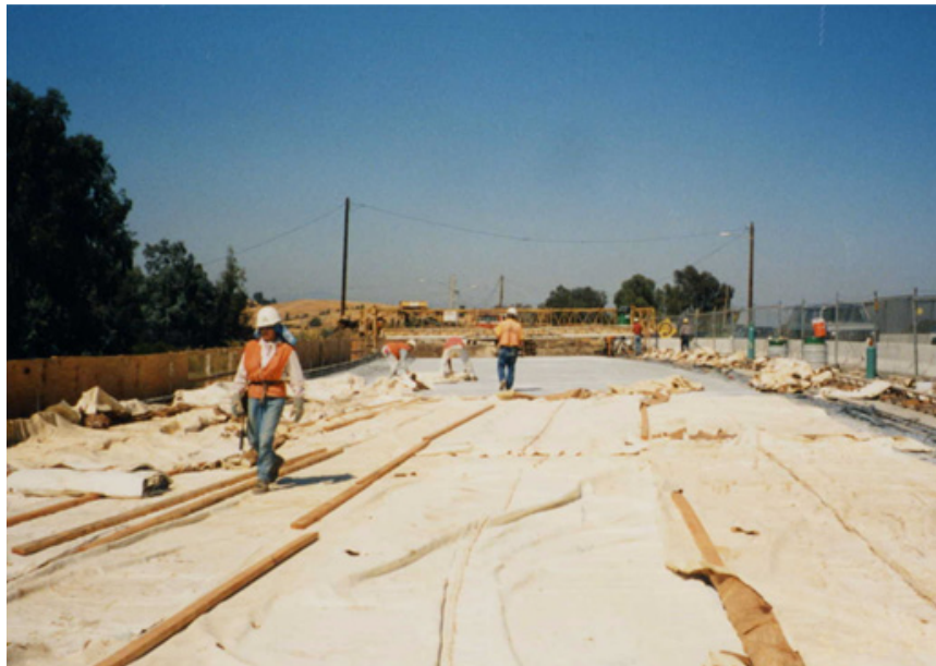
Figure 5-24. Curing with Burlene Curing Blankets.
