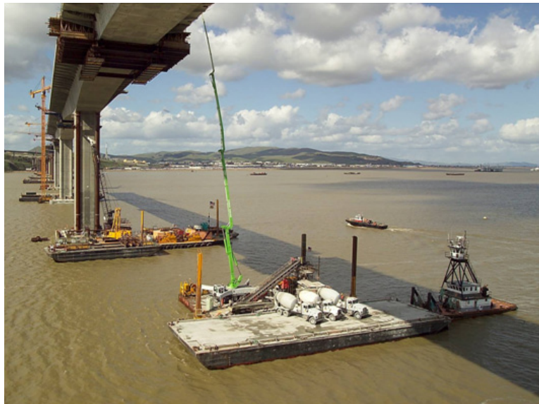
Figure 5-8. Benicia-Martinez Concrete Pumping.
