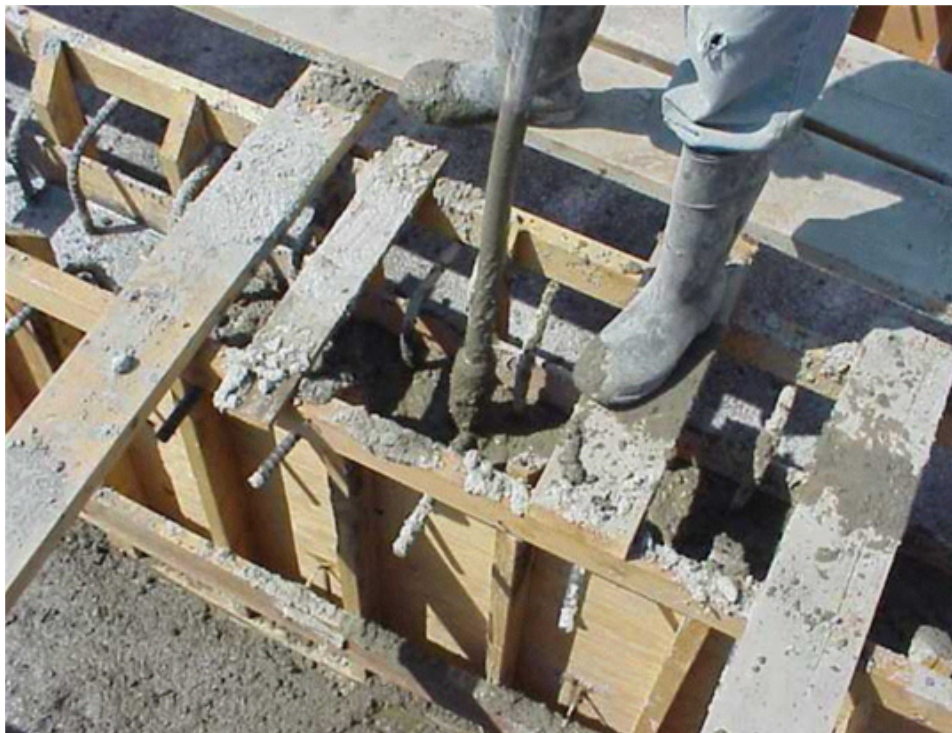
Figure 5-14. Vibrating Box Girder Stem Concrete.
