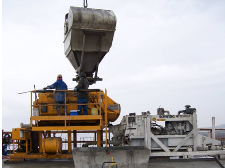
Figure 5-11. Concrete Bucket Used on the Benicia-Martinez Bridge Project.
