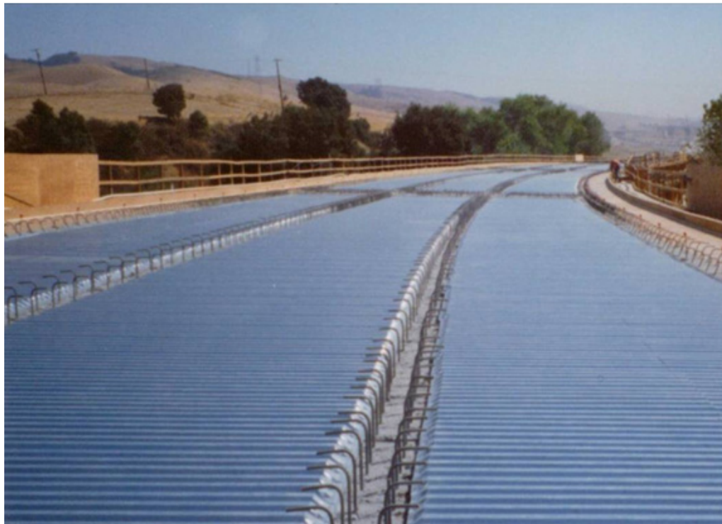
Figure 5-7. Metal Deck Forms.
