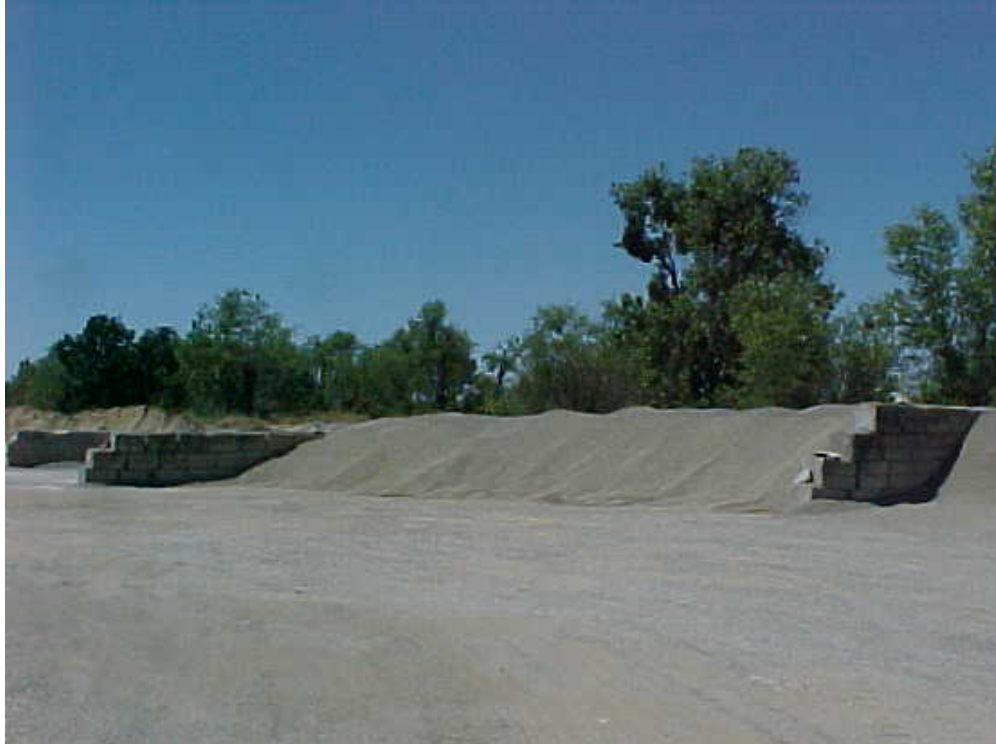
Figure 4-2. Aggregate Storage Bunkers.
