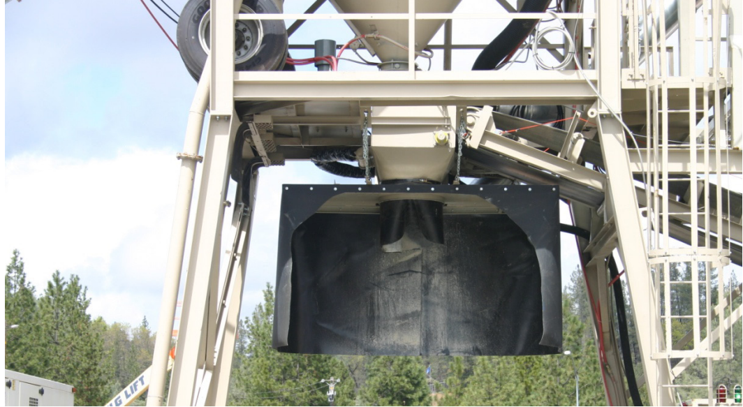
Figure 4-13. Sock Used at a Truck Mixer Charging Chute.
