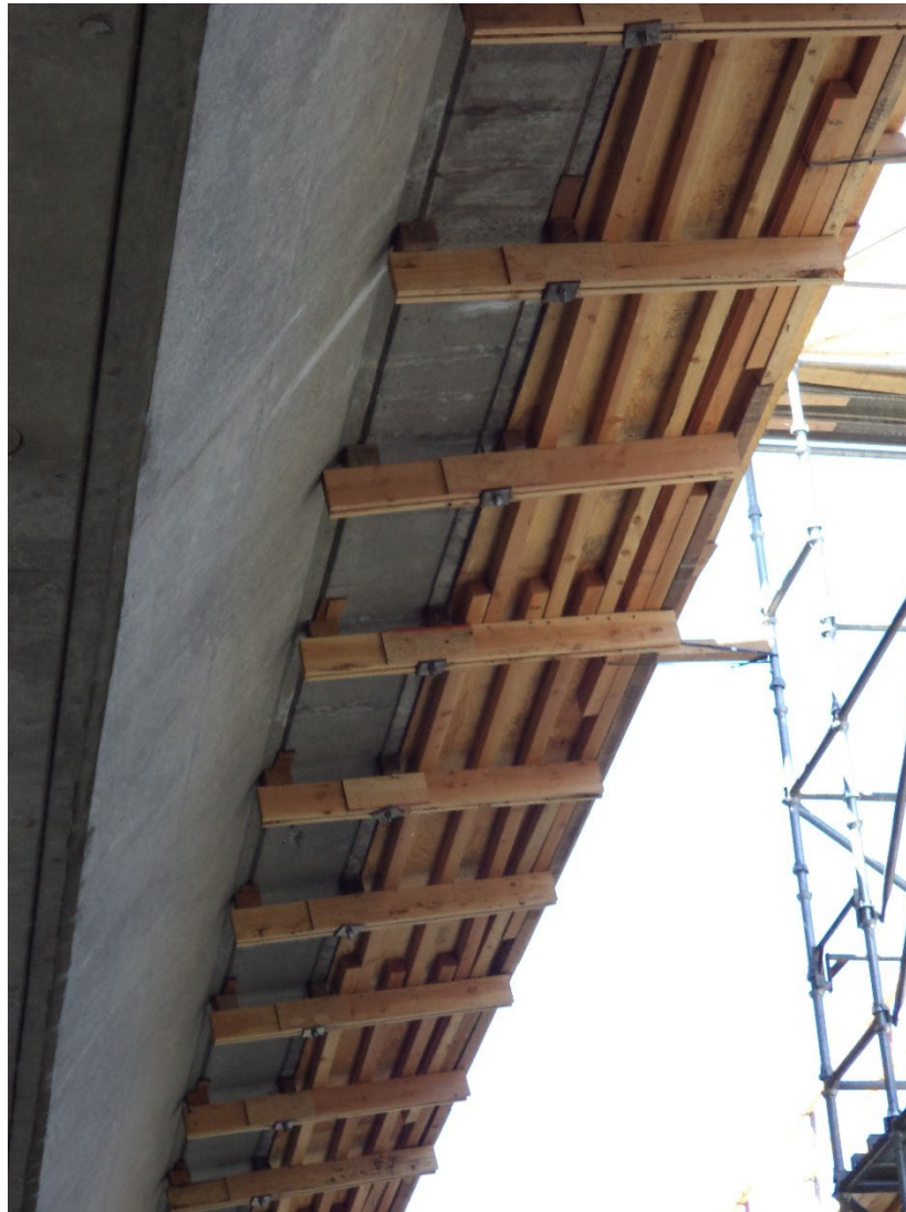
Figure 5-5. Four-Foot-Wide Protective Cover for Rail Removal, Sacramento
