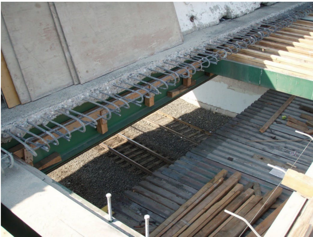
Figure 5-8. Suspended Scaffolding Over Railroad for Edge of Deck Removal, Marysville
