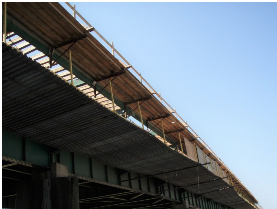
Figure 5-4. Suspended Scaffolding on Overhang for Debris Containment, Marysville
