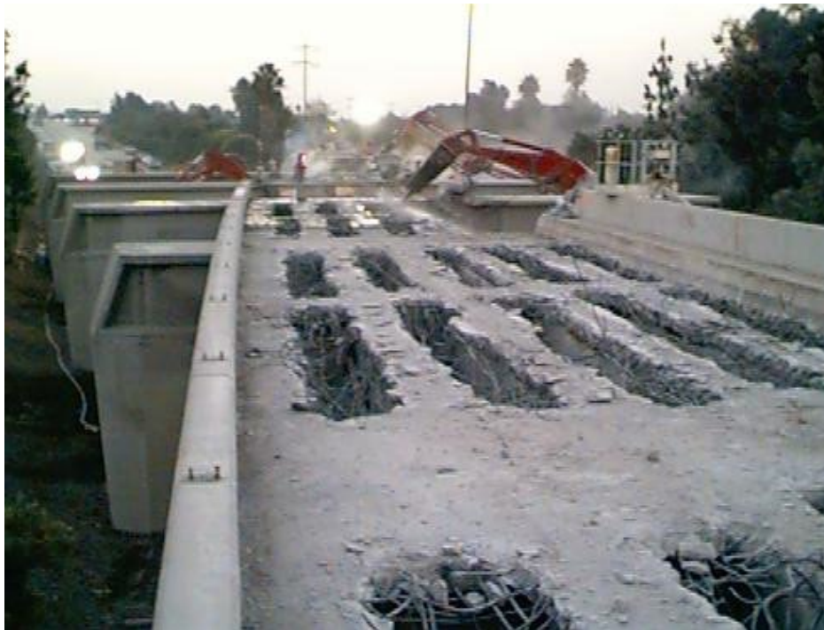
Figure 5-2. Box Girder Soffit Used as a Protective Cover, Santa Anita
