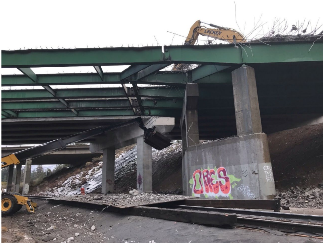
Figure 5-9. Protective Cover with Steel Plates Over Railroad, Dunsmuir
