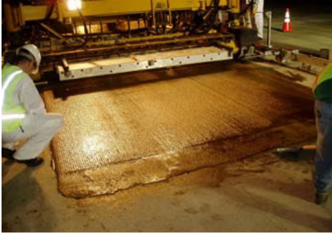
Figure 5: Trial Slab Construction
