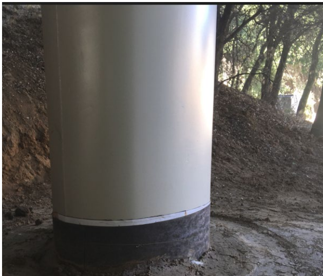
Figure 5. Waterproofing for Column Casing
