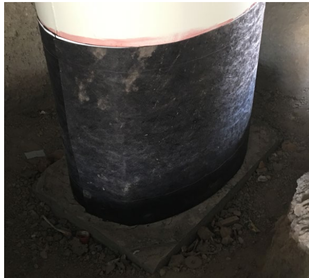
Figure 6. Waterproofing for Column Casing
