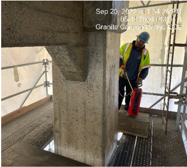
Figure 3. Applying Silane Waterproofing
