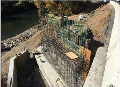
Abutment 1, Formwork Start
