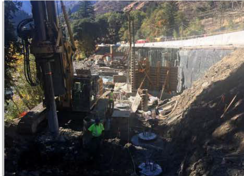
Drilling at Pier 2
