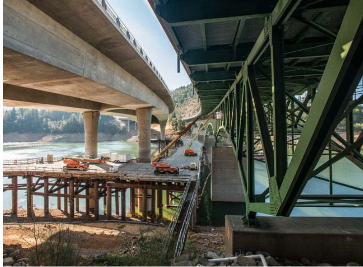
Figure 4: Structural plate steel, shown here in the bridge at right.
