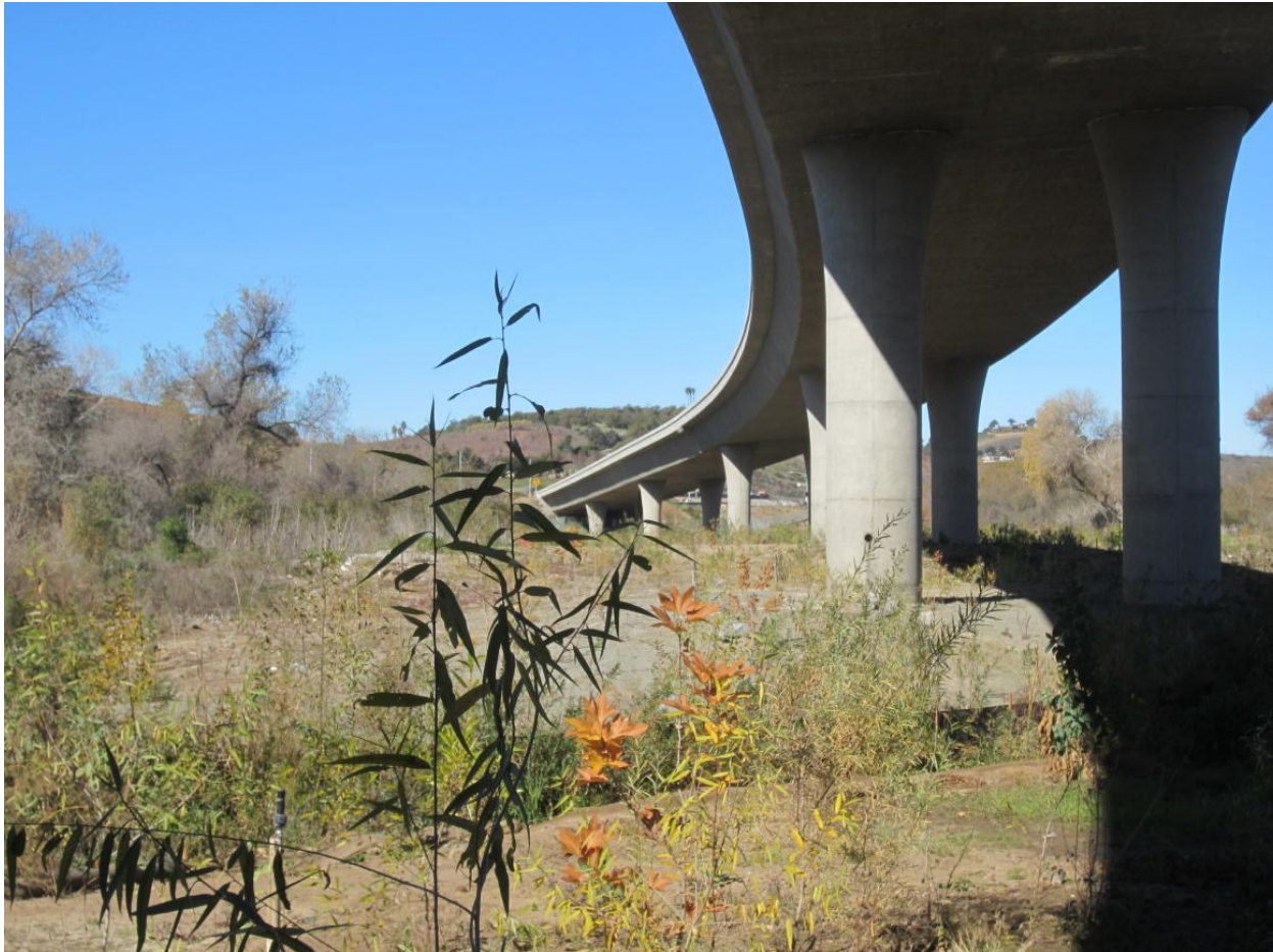
Figure 5.2.1-1 San Luis Rey River Bridge: A Concrete Box CIP/PT Bridge
